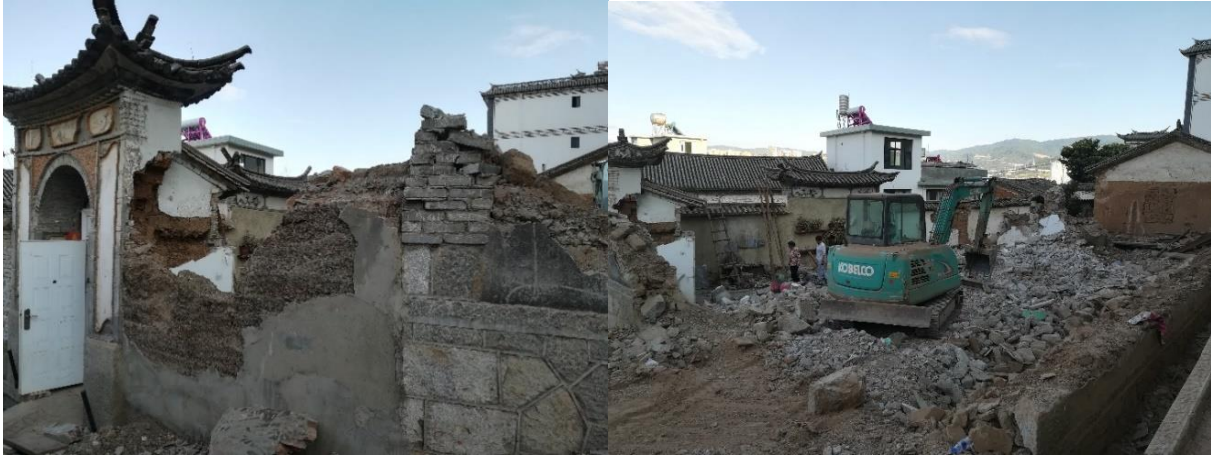
Figure 4.2.7. A construction site in a suburban village
