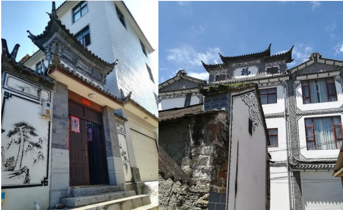
Figure 4.2.8. Modern Bai dwellings in villages
