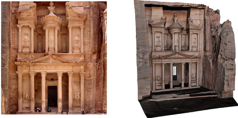
FIGURE 1.1: Photograph of Petra treasury (left), and 3D model generated from terrestrial laser scanning (right) [5].
