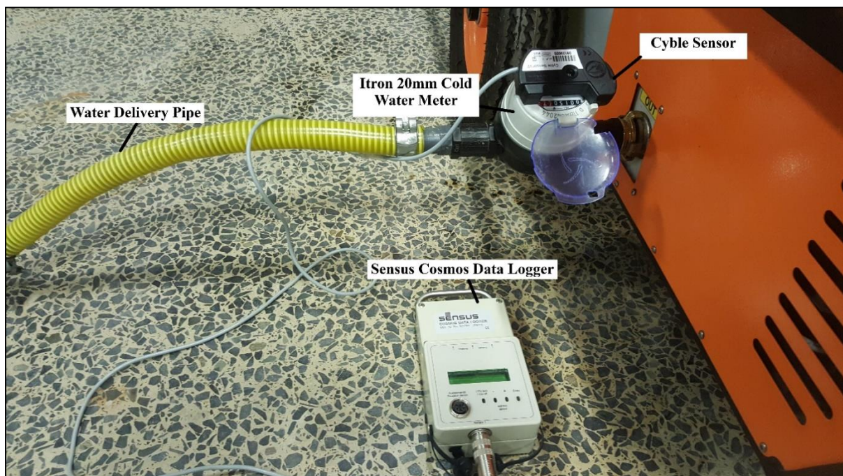
Figure 6-4 - Checking the PCAD's flow sensors
