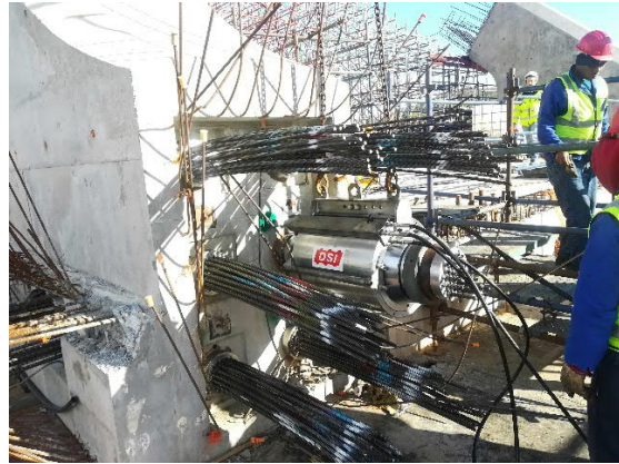
b) Ashton Arch Bridge
