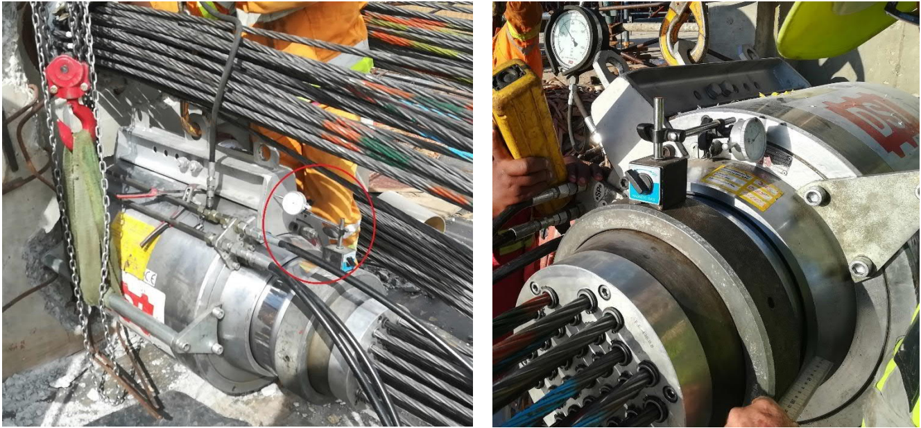
Figure 49 Jack with magnetic precision Dial Gauge
