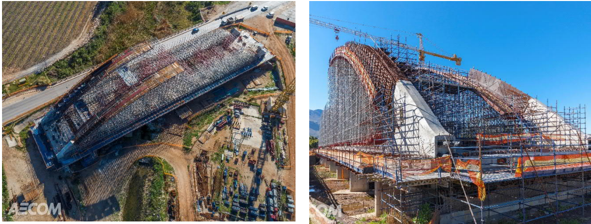
Figure 2 Ashton Arch Bridge during construction. Photographed by Terry February for AECOM, 2018.
