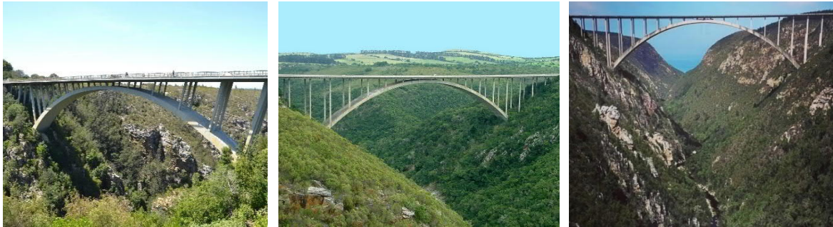
a) Paul Sauer Bridge (1956) b) Van Stadens Bridge (1971) c) Bloukrans Bridge (1983)
