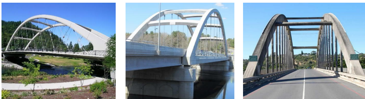
a) Depot Street bridge (2006) b) Covered Bridge (2012) c) Nico Malan bridge (1971)
