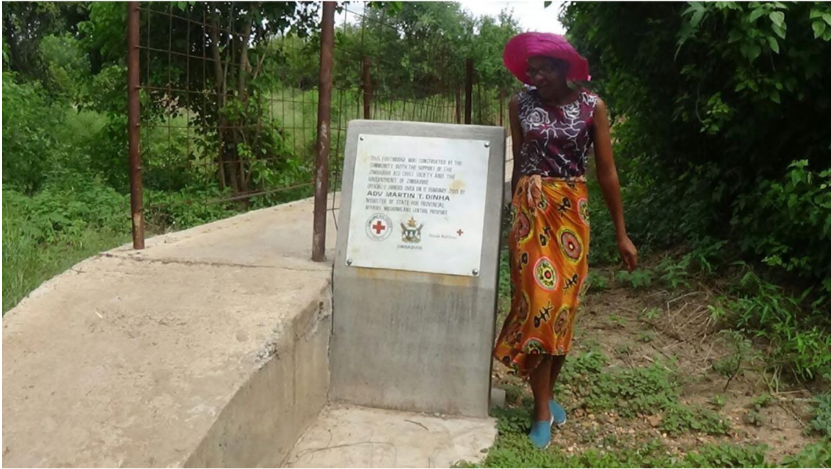
The researcher at the footbridge that was constructed by Chadereka community members across Nzoumvunda River.
