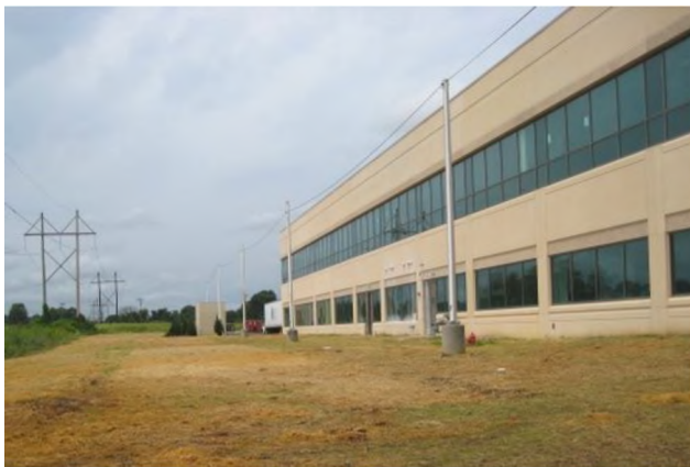
Figure 4.6 ELF EMF radiation Active shielding installation EMF Services, 2015)
