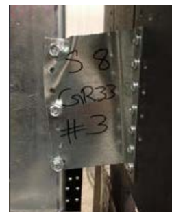
(b) local buckling failure
