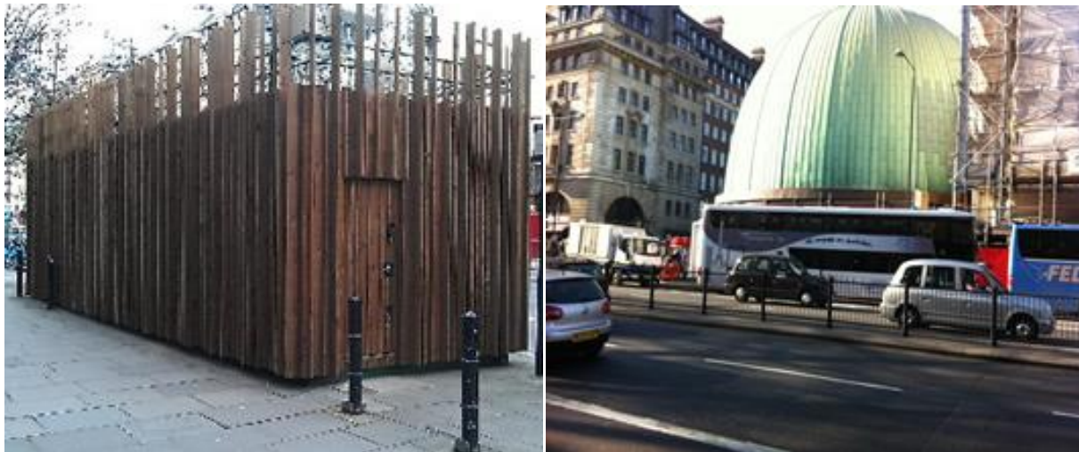
Figure 2.4 Marylebone Road AURN Station (left) and the view from the North (right). Reprinted with permission from the Department for Environment Food & Rural Affairs. (237)
