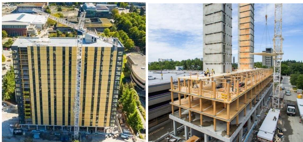
Figure 2.18 UBC's Brock Commons Buildings, Canada (UBC News 2016)
