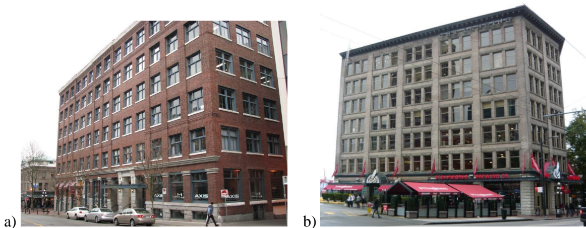
Figure 2.4 Old tall wood buildings in Canada: a) Leckie Building; b) The Landing (Koo, 2013)
