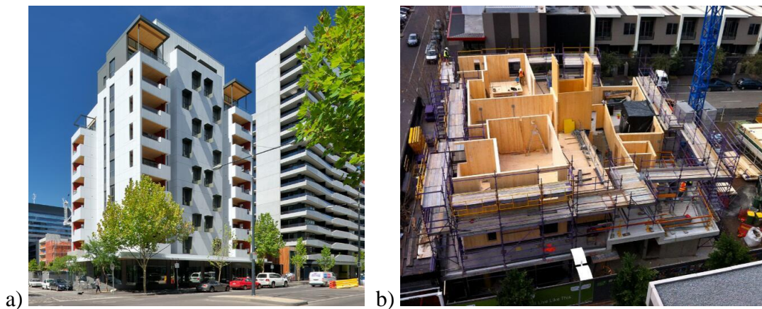
Figure 2.9 Forté Building, Australia: a) Overview; b) Construction (victoriaharbour.com.au)
