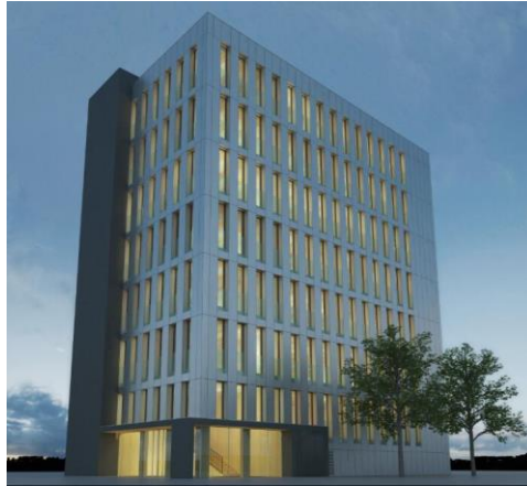
Figure 2.15 Lifecycle Tower One, Austria (engineering.com)
