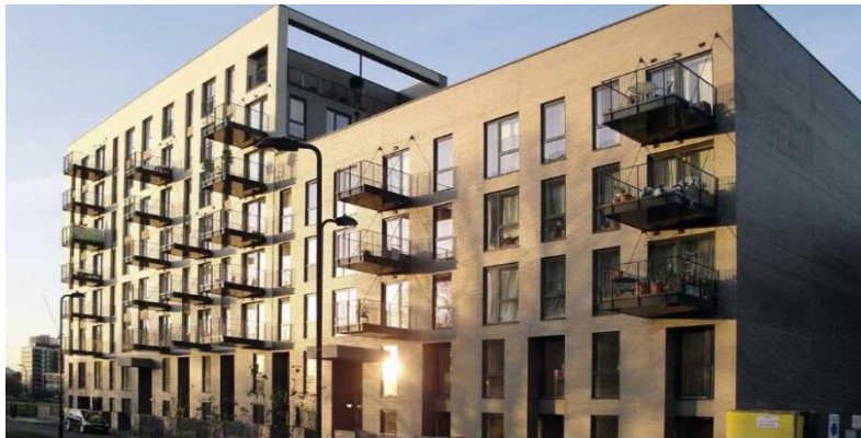
Figure 2.8 Bridport House, UK (peterbrett.com)
