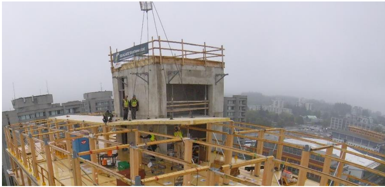
Figure 43: Fit CLT into location
