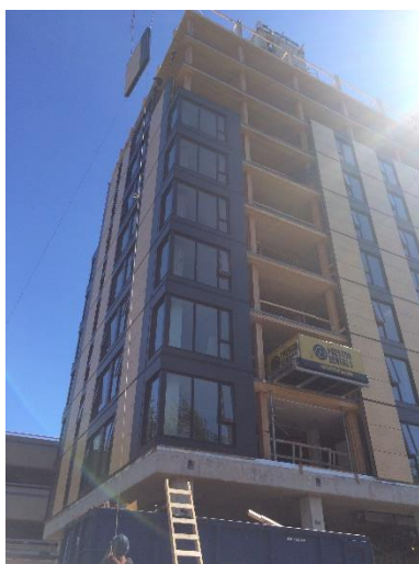
Figure 46: Installation of envelope panels
