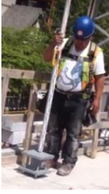
Figure 38: Pedestal elevation check
