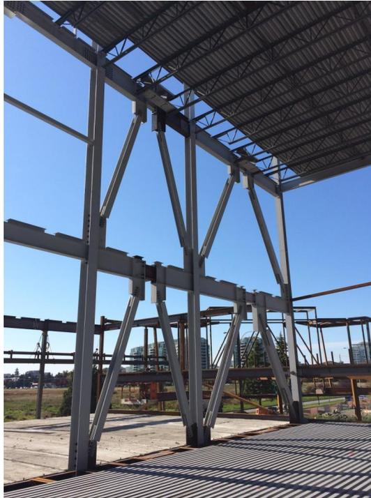
**Figure 4.** REBF systems using bolted link in Richmond B.C. (2016)
