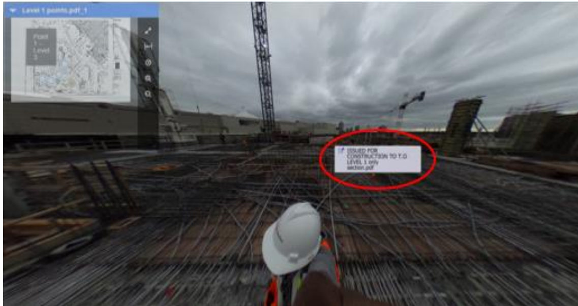
Figure 6.20: Sample image highlighting how the relevant project documents can be embedded within spherical images which can then be used efficiently during future facilities management.
