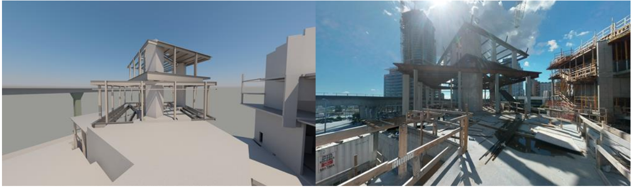
Figure 6.11: Design compliance review conducted directly by comparison with the spherical image generated from the design BIM.
