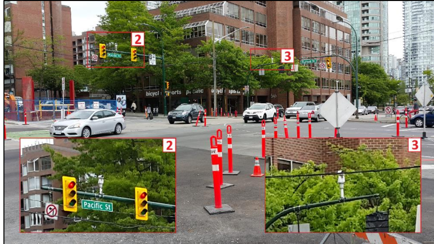
Figure 3-8: Location of cameras 2 and 3 (as seen from the West traffic island).
