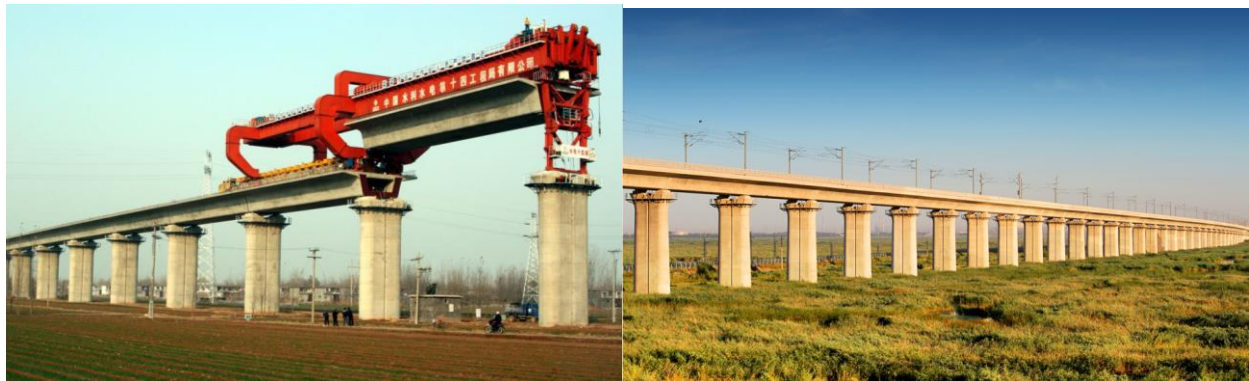
Figure 1 Typical HSR MSSS bridges in China (Authorized by Huitu.com)
