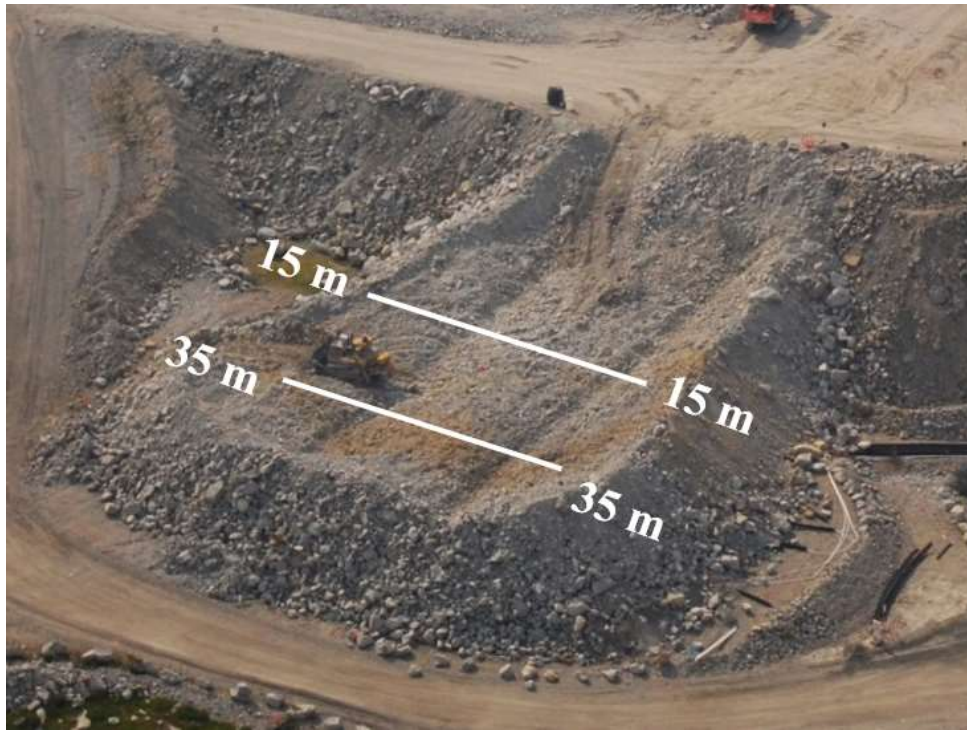
Figure 2.7. Approximate positions of the 15 m and the 35 m sampling lines across the partially deconstructed Type I pile (Atherton, 2017).
