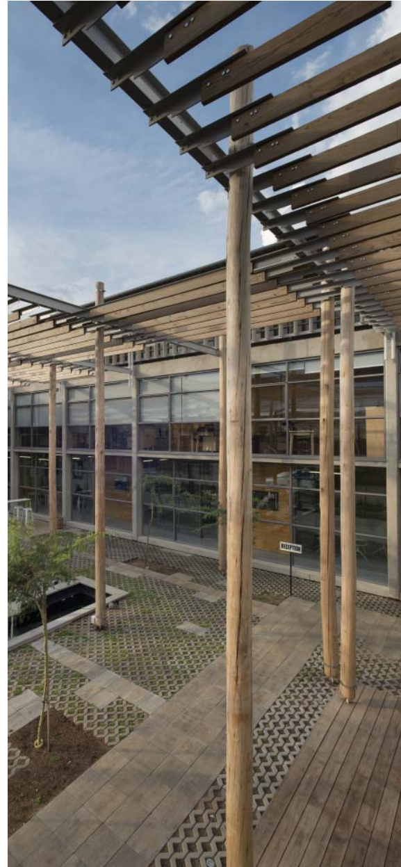
Figure 7.12: View of Southern courtyard and pergola structure indicating the honesty and simplicity of materials expressed through detail connections (Source: DOOK Photography, n.d., adapted by Author). http://images.adsttc.com/media/images/578d/8345/e58e/ce05/ed00/0058/large_jpg/I-Cat__AfriSam_Dook_24.jpg?1468891937
