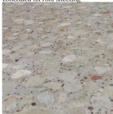
polished concrete floor
