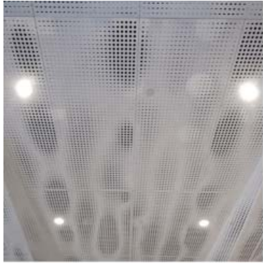
perforated steel ceiling
