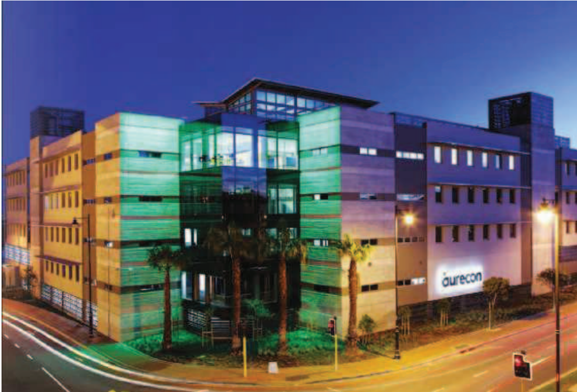
IMAGE 4.8: The Aurecon Building in Century City, South Africa's first Green Star South Africa Five Star rated building (Rabie Property Group & Century City Property Owners' Association, 2015: 12).
