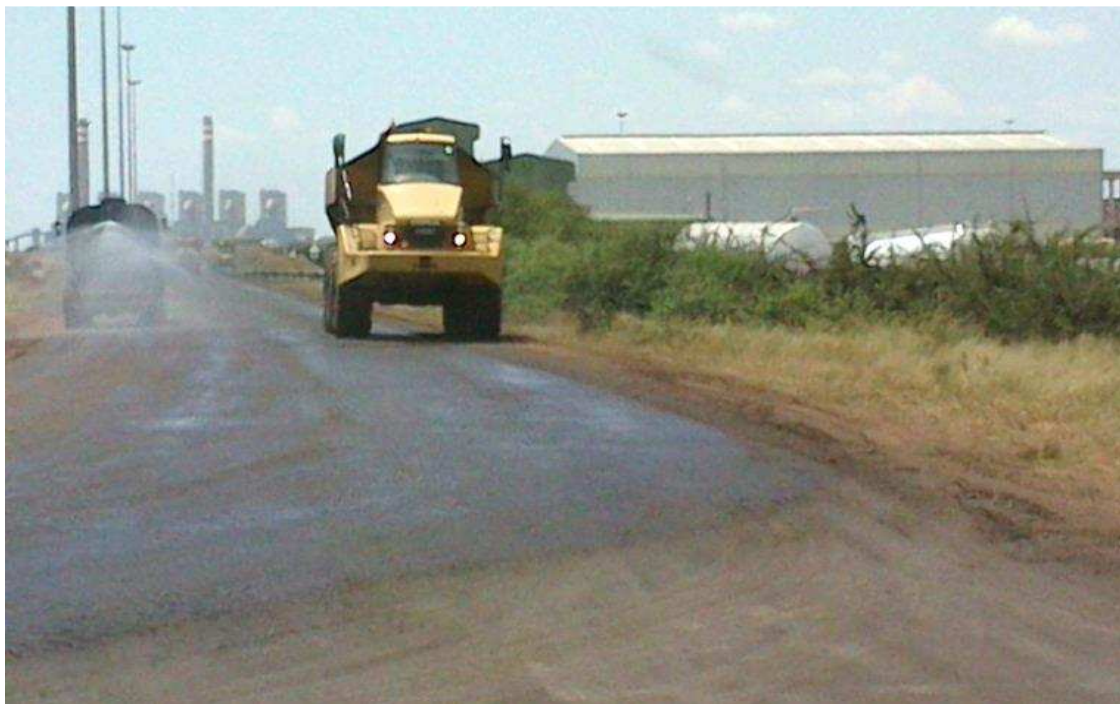
Figure 4.13 Dust suppression at Medupi
