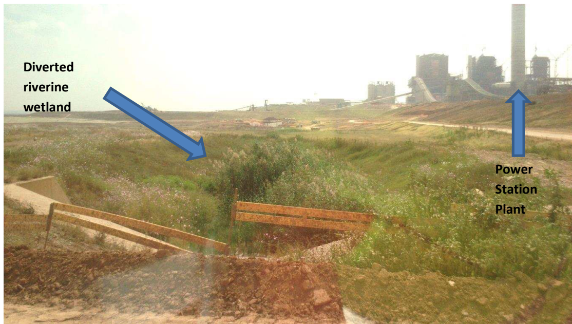
Figure 1.2 Diverted riverine wetland within Kusile construction site
