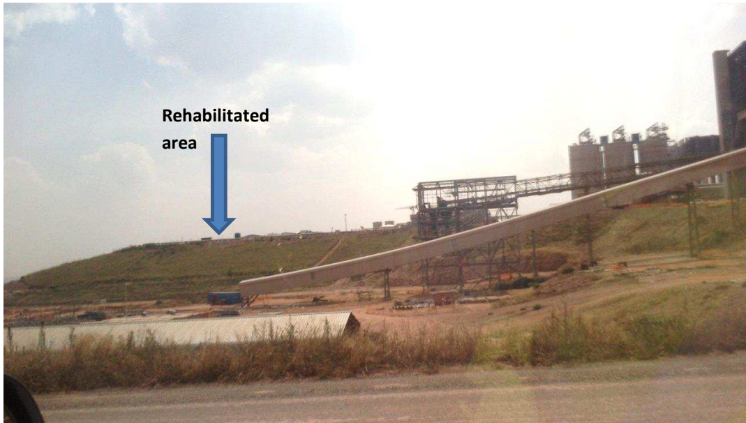
Figure 4.8 Rehabilitation of some area at Kusile
