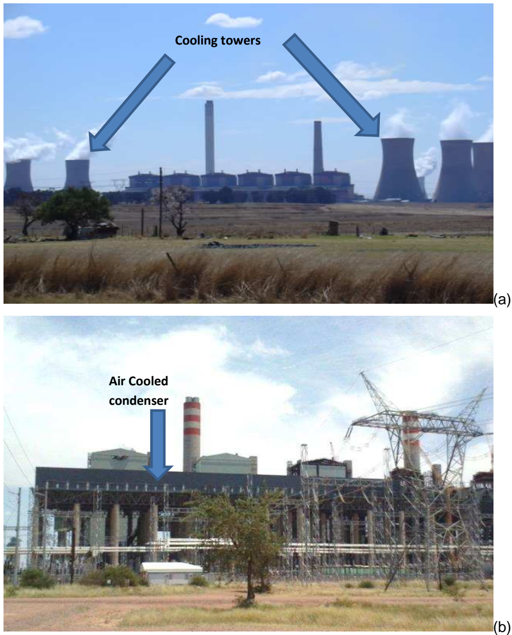
Figure 4.16 Power stations cooling structures (a) normal cooling towers structure and (b) Medupi air cooled condenser structure.
