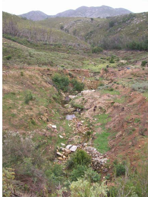
Figure 3.7: A damaged tributary in the Kromme River. The headcut moved backwards up the hill, eroding away sediment and vegetation
