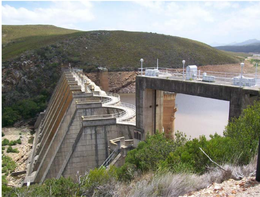
Figure 3.18: The multi-arched Churchill Dam on the Kromme River in the Eastern Cape of South Africa
