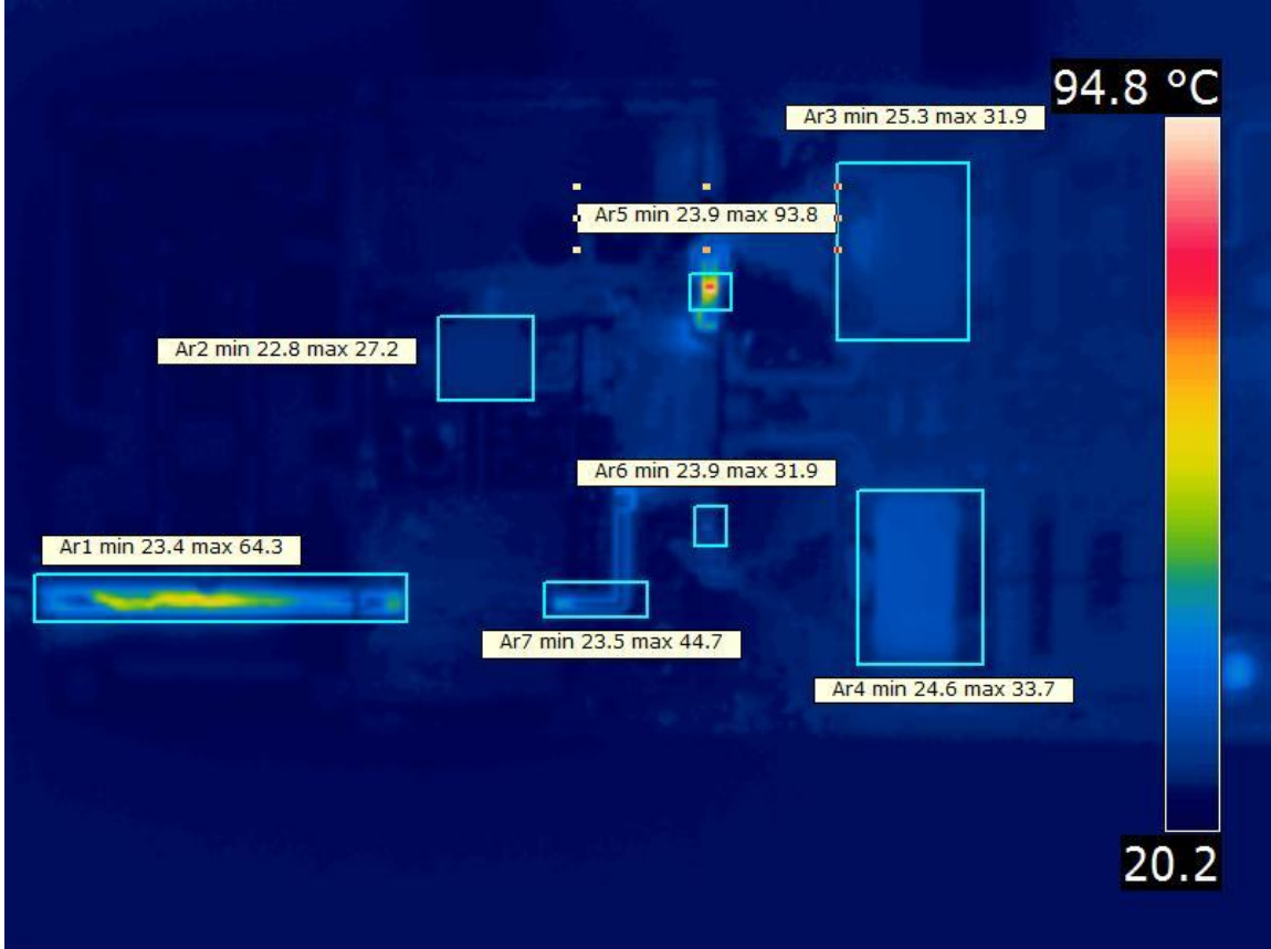
Figure 64. IR picture at 100 watts of power input.
