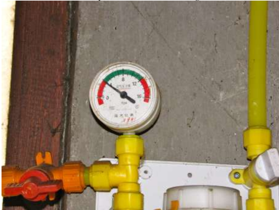
Picture 2.2, pressure meter before biogas stove
