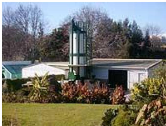
Photograph 2.4: A vertical composting reactor
