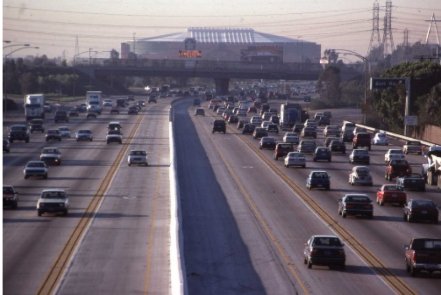
Figure 10. Example of concurrent flow lanes in California.
