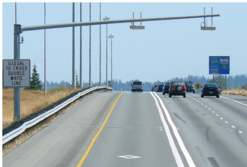
Figure 43. Toll reader gantry on SR 167 in Seattle, Washington.
