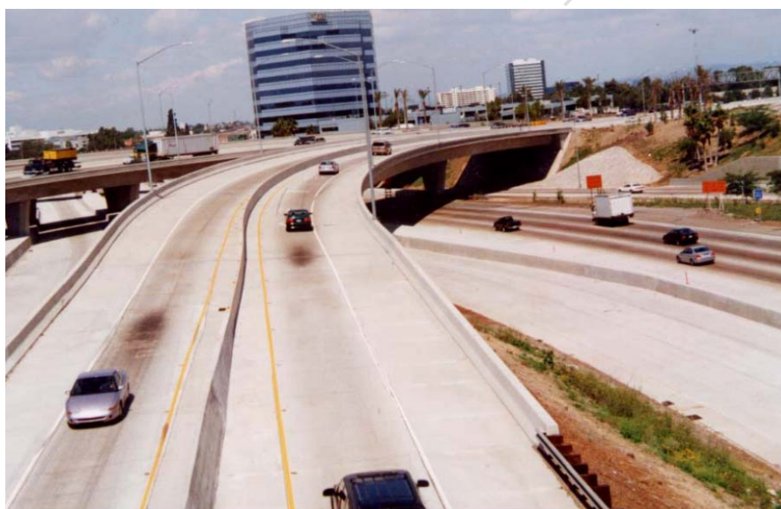
Figure 58. Two-way interchange flyover ramp.
