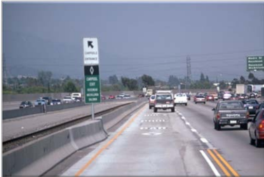
Figure 86. Example of pavement markings at a roadside geometric impediment within a tangent section.
