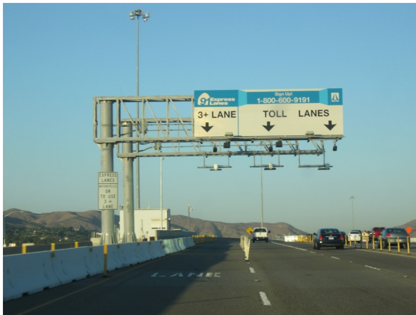
Figure 44. Toll beacons located on back side of gantry on I-15 in San Diego, California.
