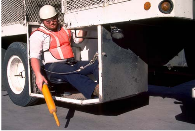
Figure 78. Deployment of contraflow lanes by pylons.
