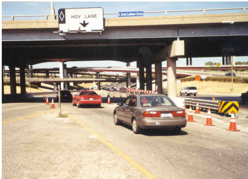
Figure 79. Typical median crossover on a contraflow lane on I-30 in Dallas.
