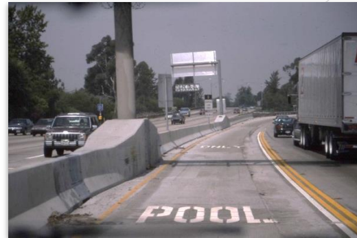
Figure 87. Example of pavement markings at a roadside geometric impediment within a horizontal curve section.
