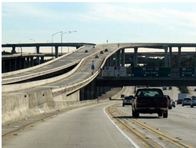
Figure 54. Ground-level view of direct-access managed lane ramp in Houston, Texas.
