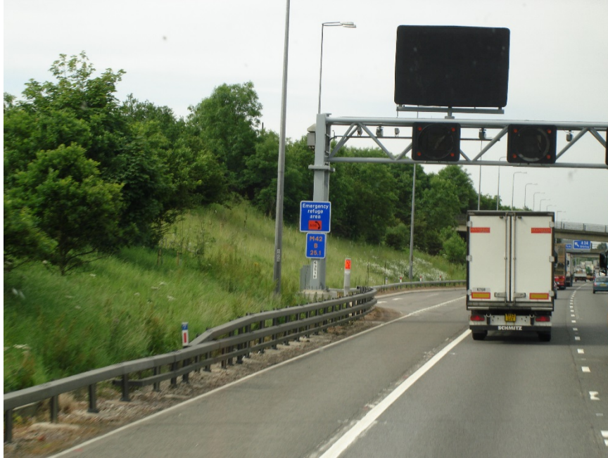
Figure 40. Driver's view of approach to emergency refuge area in England.
