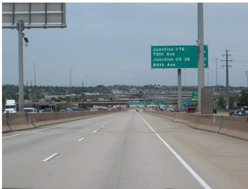
Figure 30. Example of barrier-separated managed lane on I-25 in Denver, Colorado.
