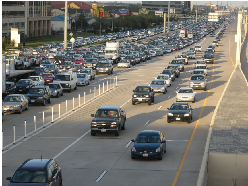
Figure 32. Example of pylons separating managed lanes from general-purpose lanes on the Katy Freeway (I-10) in Houston, Texas.
