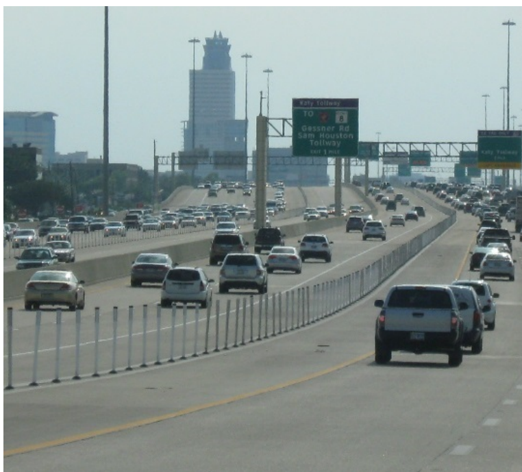
Figure 11. Example of roadway separated by pylons on I-10 in Houston.
