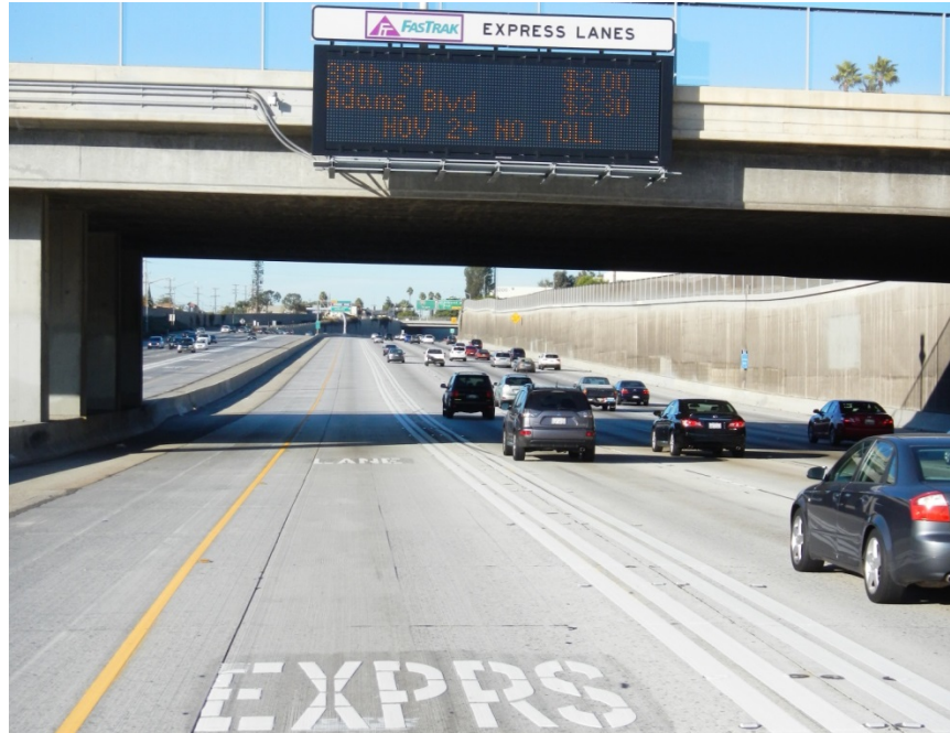
Figure 31. Example of buffer-separated managed lane on I-110 in Gardena, California.
