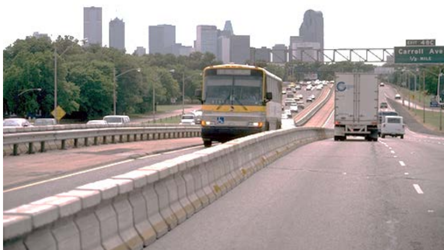
Figure 16. Example of contraflow lane in Dallas.
