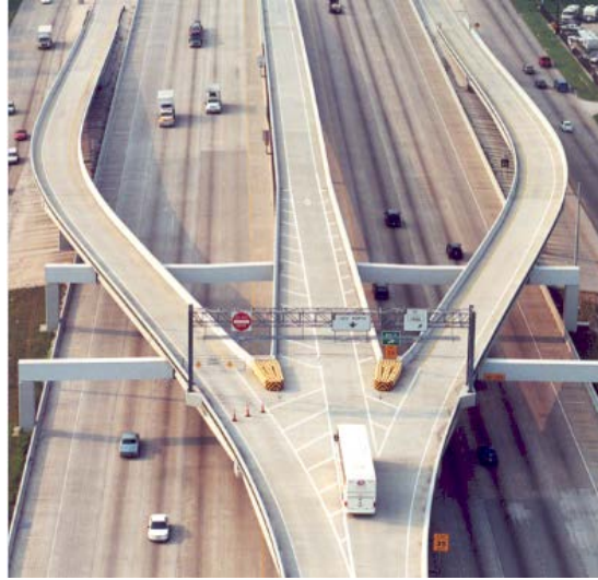
Figure 52. Example of direct-access managed lane ramps over general-purpose lanes in Houston, Texas.
