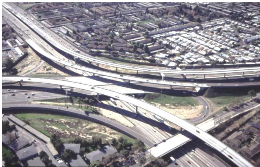
Figure 57. Aerial view of two-way interchange flyover ramps.
