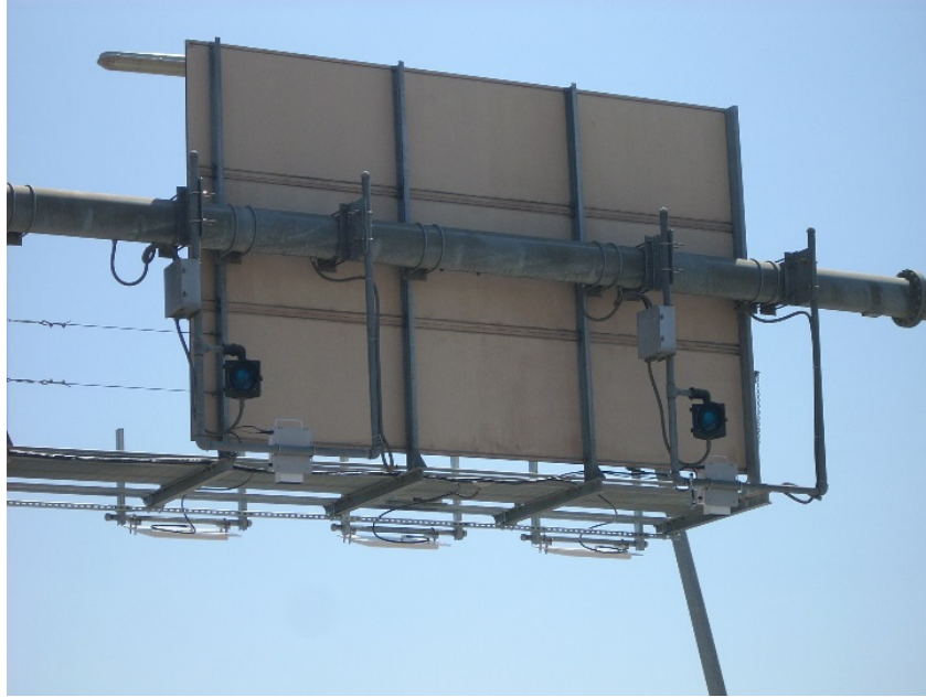
Figure 44. Toll beacons located on back side of gantry on I-15 in San Diego, California.
