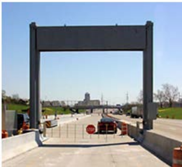
Figure 75. Tower vehicle-arresting device in place when the managed lane is closed.
