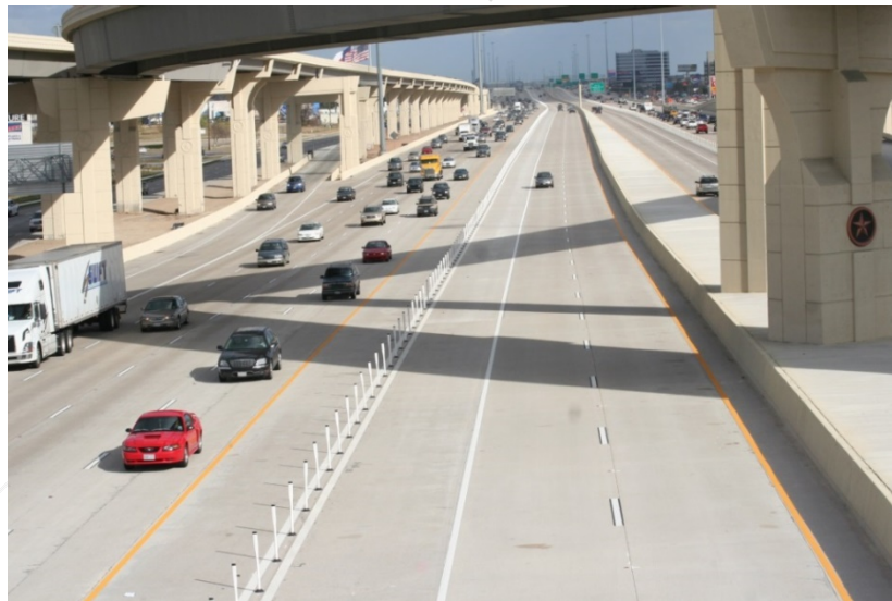
Figure 61. Managed lanes with available width for future enhancements on US-290 in Houston, Texas.
