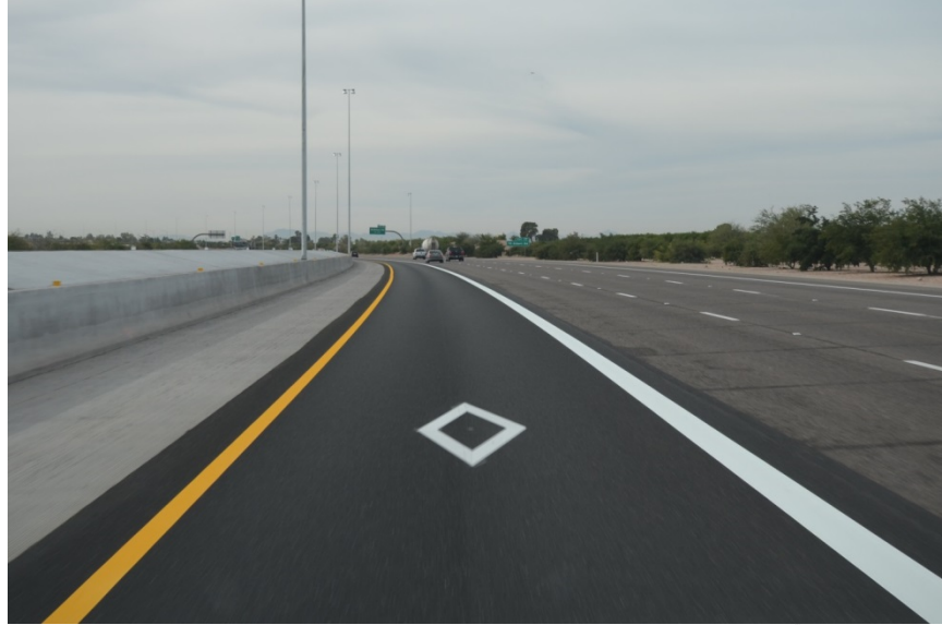
Figure 33. Example of pavement marking separation on Arizona Loop 202 in Maricopa County, Arizona.
