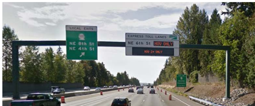
Figure 71. Variable occupancy messages displayed on CMS over HOV lane on I-405 Express Lanes in Seattle.
