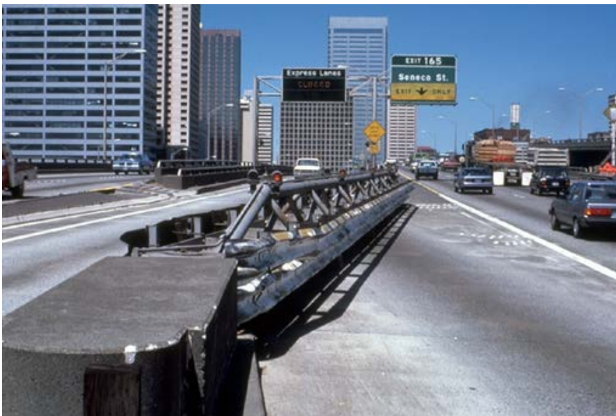
Figure 13. Graphic example of reversible-flow median lane.
