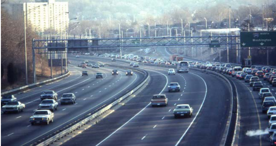
Figure 12. Example of reversible lanes on I-395 in Virginia.
