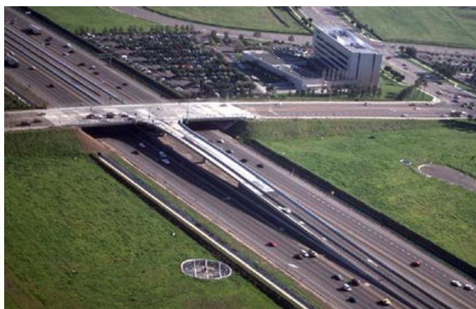
Figure 55. Example of direct-access managed lane ramp to local street in Houston, Texas.
