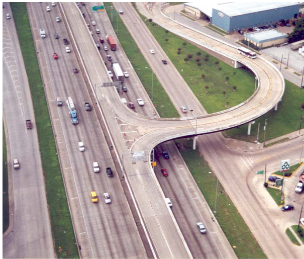
Figure 53. Example of direct-access managed lane ramp to park-and-ride facility in Houston, Texas.
