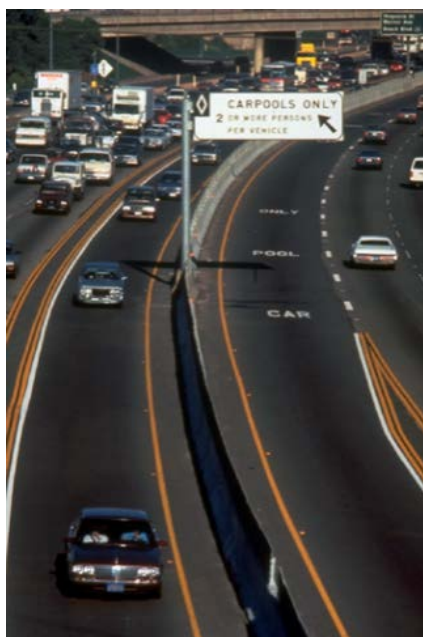
Figure 23. Typical HOV lane access in California.
