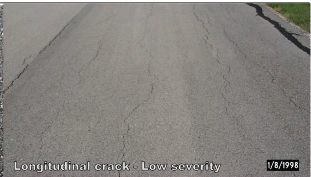
Longitudinal cracking - Low severity
