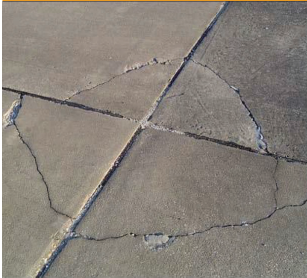
Corner Break - Low severity
