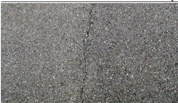
Longitudinal crack - Low severity
