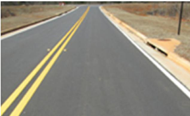
FIGURE 29 Look of high RAP pavements after implementation of the corrected optimum asphalt content (Source: Hines 2015).
