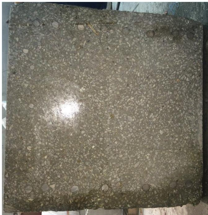
**Figure 2-42.** Saw cut at the middle of bridge pier cap.
