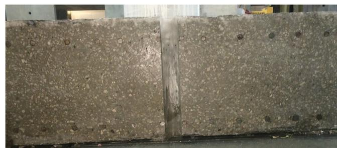
**Figure 2-40. Saw cut at the middle of the bridge pier footing.**
