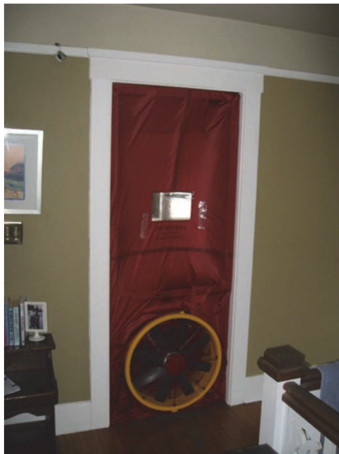
Figure 4-9. Blower door test.
