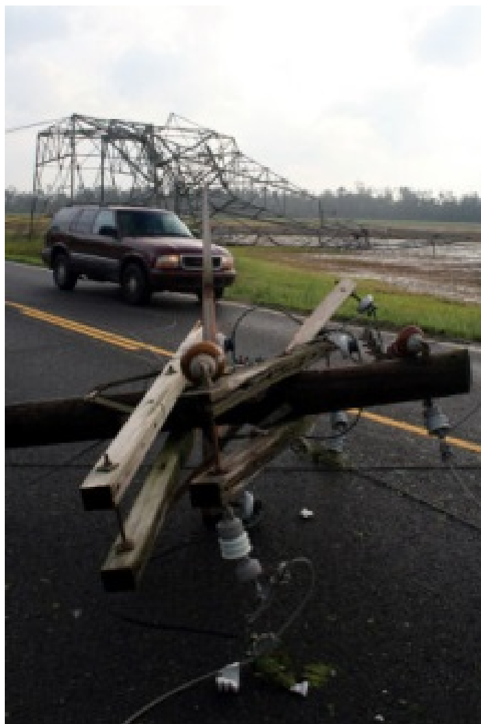
FIGURE 7.4 An example of transmission (background) and distribution (foreground) electrical infrastructure damage associated with the 2008 Hurricane Gustav in southern Louisiana. SOURCE: Entergy, “Images – Gustav Damage,” image gallery, http://www.entergy.com/2008_hurricanes/gustav_media.aspx . Courtesy of Entergy.
