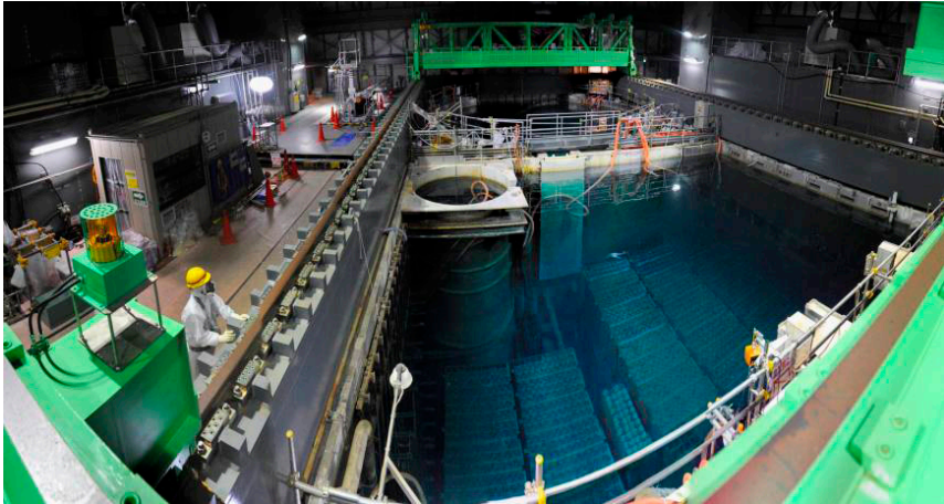
FIGURE 2.5 Photo of the Unit 4 refueling deck at the Fukushima Daiichi plant taken on November 7, 2013. Notes: The spent fuel pool is shown in the foreground; the fuel racks are visible at the bottom of the pool. The reactor well (background) is separated from the pool by the steel gate shown on the far wall of the pool. The green apparatus located above the reactor well is used to lift the gates and runs along tracks on the sides of the pool. The green apparatus that is partially visible in the foreground is the fuel handling machine. It also runs along tracks on the sides of the pool. The photo is distorted because it was taken with an ultra-wide-angle lens. SOURCE: Kyodo News.
