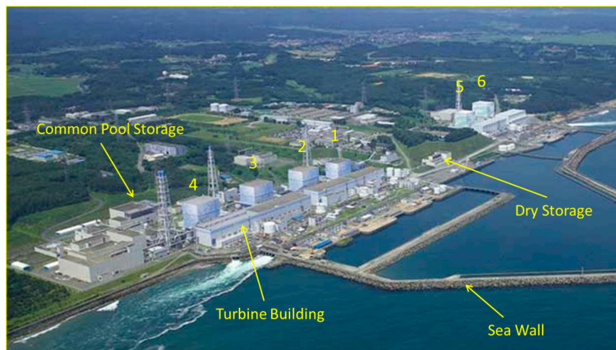
FIGURE 2.1 Oblique aerial photo of the Fukushima Daiichi Nuclear Power Station prior to the March 11, 2011, earthquake and tsunami. Note: Spent fuel was being stored in the Unit 1-6 reactor buildings, the common pool, and in a dry cask storage facility. SOURCE: Photo courtesy of TEPCO.
