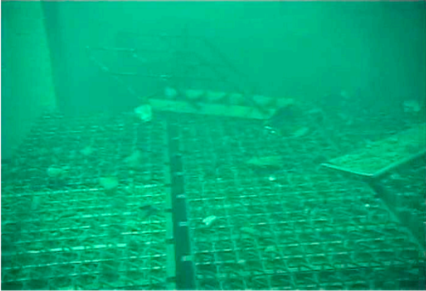
FIGURE 2.11 Debris on top of fuel racks in Unit 4 pool. SOURCE: TEPCO (2012a, Attachment 9-5, Figure 7).
