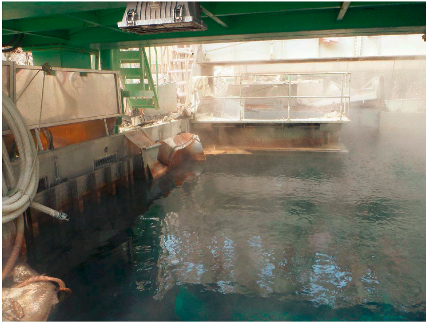
FIGURE 2B.2 Water evaporating from the surface of the Unit 4 spent fuel pool. SOURCE: TEPCO image released June 29, 2011.
