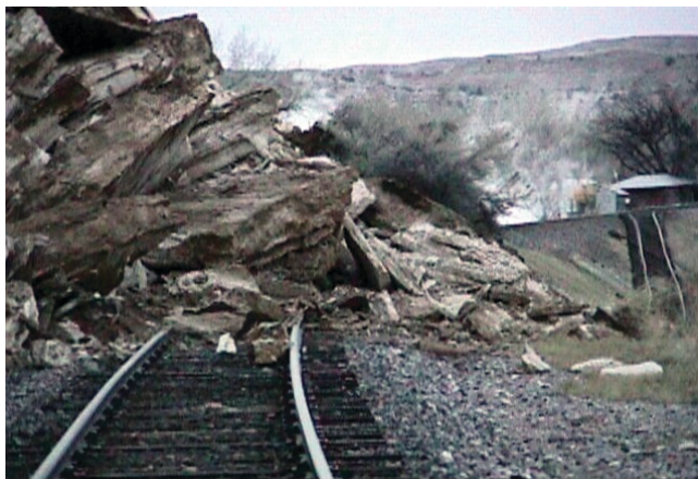
FIGURE 3 Rockfall, Thermopolis, Wyoming, 2002. (Photo credit: D. McCulloch.)
