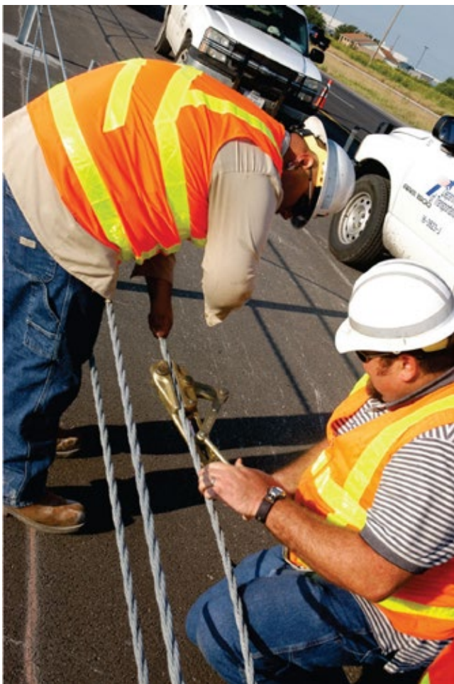
FIGURE 11 2012 Texas DOT Contraflow Evacuation Exercise—Cable barrier removal (Courtesy: TxDOT).
