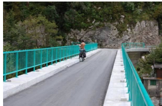
Čezsoški Bridge, Slovenia, after application of UHPFRC. (Source: ARCHES report.)
