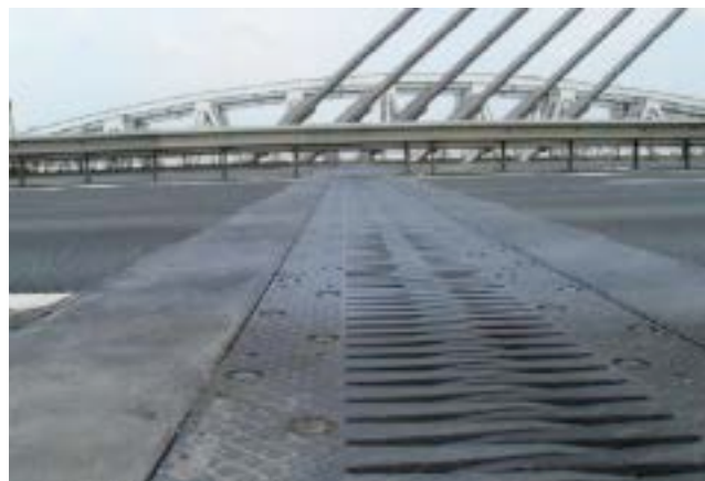
FIGURE 8 Expansion joints.
