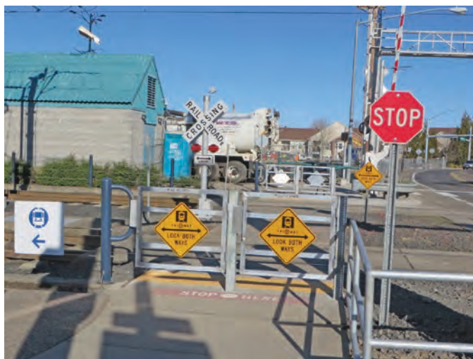
Figure 130. Example of swing gates with a STOP sign.
