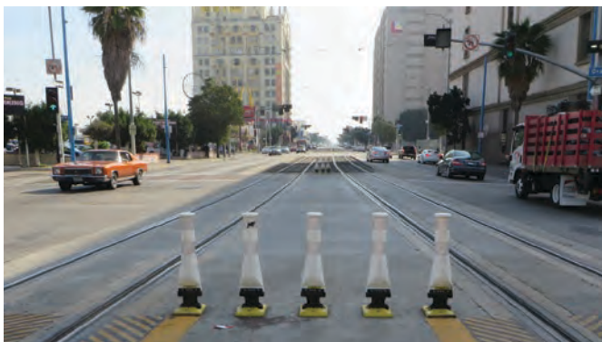
Figure 61. Closeup of flexible bollards on the end of the station.
