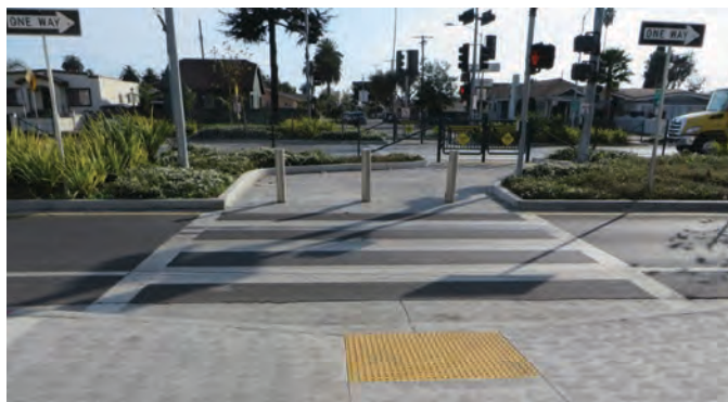
Figure 46. Landscaping channelizes pedestrians to the appropriate crossing location while the detectable warning at the bottom of the curb ramp is a good cue for visually impaired pedestrians that they have reached the edge of the street and are at a crosswalk.
