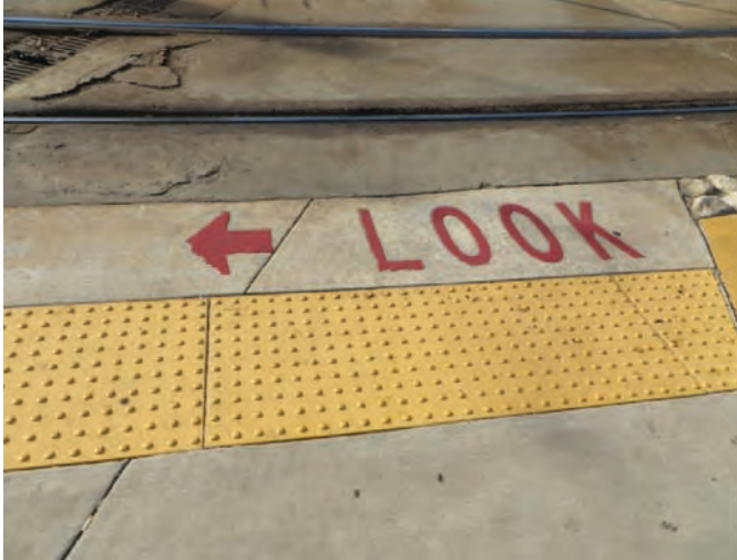
Figure 111. LOOK pavement markings near detectable warning in Baltimore.
