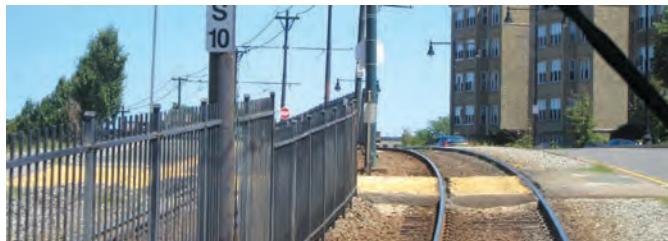
Figure 37. Example of a change in fence height prior to pedestrian crossing to improve sight distance.
