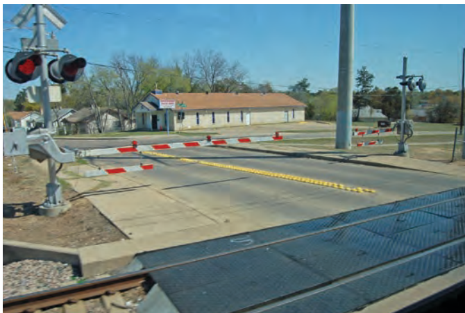
Figure 129. Example of a horizontal hanging bar on a vehicle gate arm at a DART crossing.
