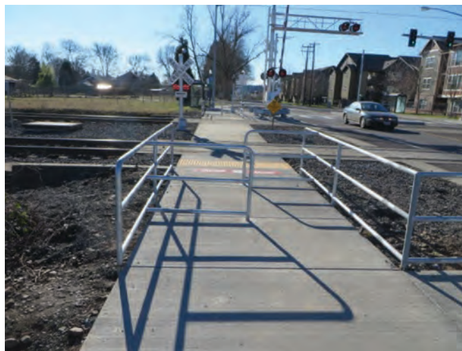
Figure 35. Example of tubular barriers used to slow pedestrians.
