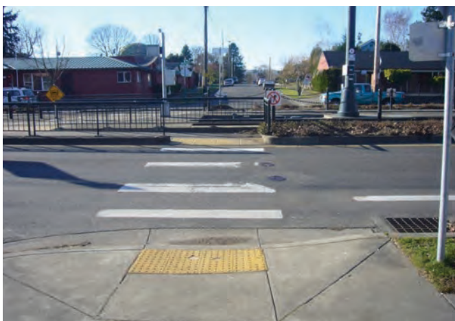
Figure 45. The channelizing fencing guides pedestrians who are visually impaired to the intended crossing location.
