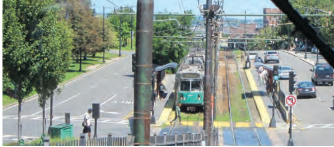
Figure 9. Example of pedestrian-rail crossing at a station adjacent to a motor vehicle crossing for median-running light rail in Boston.
