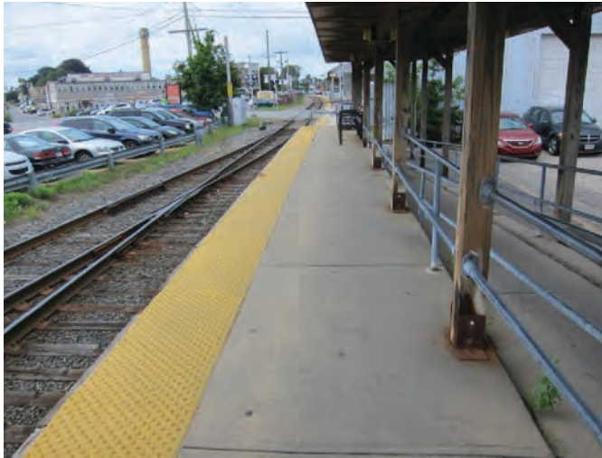
Figure 106. Example of a yellow detectable warning strip used at the edge of a platform.
