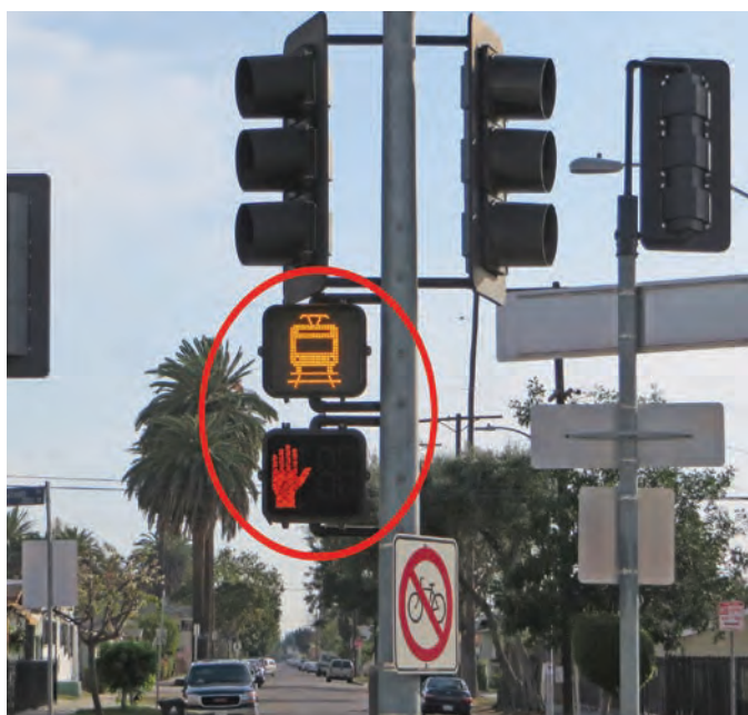
Figure 92. Example of train blank-out signs mounted above the pedestrian signal head.
