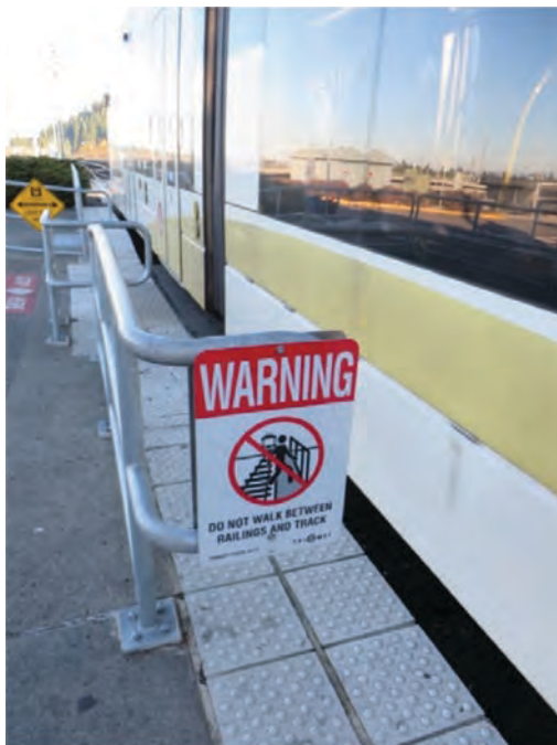
Figure 29. Example of a handle used to restrict movement between the pedestrian walkway and tracks/train.
