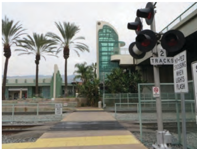
Figure 38. In-station pedestrian crossing where fencing is used to restrict crossing to a designated location.
