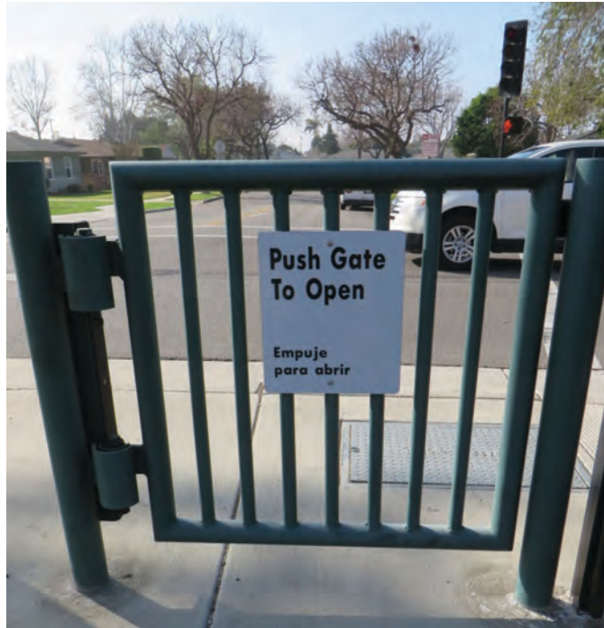
Figure 133. Example of a swing gate for emergency exit from the rail side (note that a kick plate should be present).
