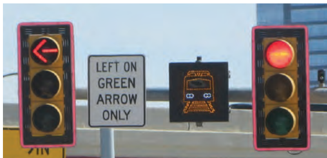
Figure 100. Example of red back plates added to signal heads to help reinforce the stop message in Houston (the mast arm also includes a blank-out sign showing a train).
