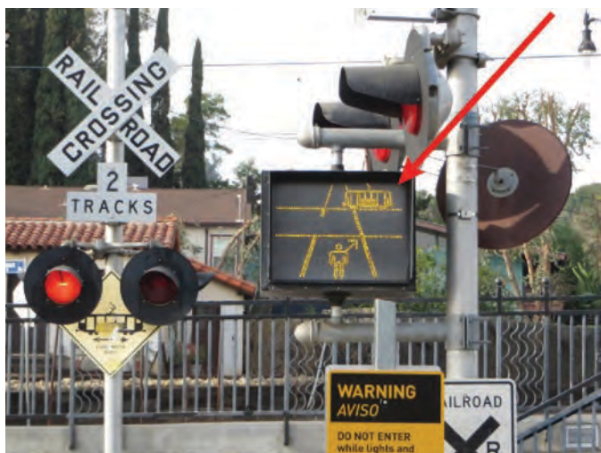
Figure 91. The pictogram within this blank-out sign in Los Angeles shows a side view of trains approaching from the right.
