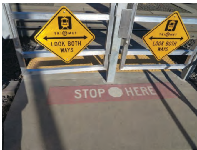
Figure 103. Example of STOP HERE pavement marking in conjunction with a swing gate in Portland.
