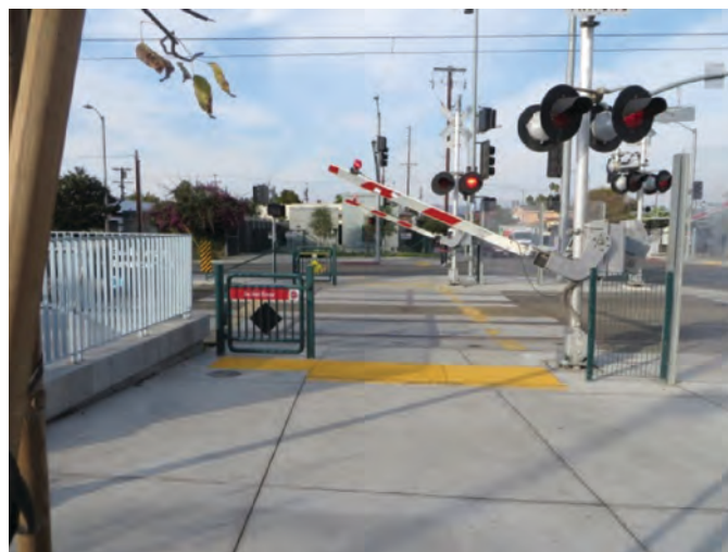
Figure 108. Detectable warnings installed across a sidewalk at an automatic gate arm on the side opposite the tracks.
