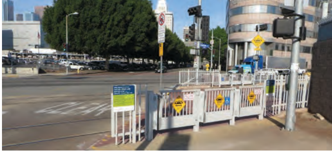
Figure 131. Examples of swing gates used at a pedestrian crossing near a station in Los Angeles.
