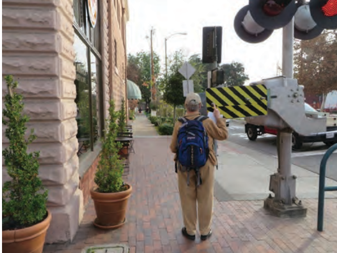
Figure 14. Example of conflict between a pedestrian and a counterweight. The pedestrian's finger is resting on a bolt that protrudes 1 inch, at her eye height.
