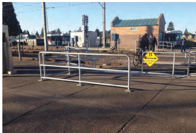
Figure 174. Pedestrian channelization at a MAX platform crossing.
