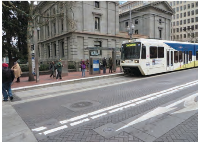
Figure 112. Example of using smooth concrete for the train as compared to the brick pattern in the neighboring lanes.
