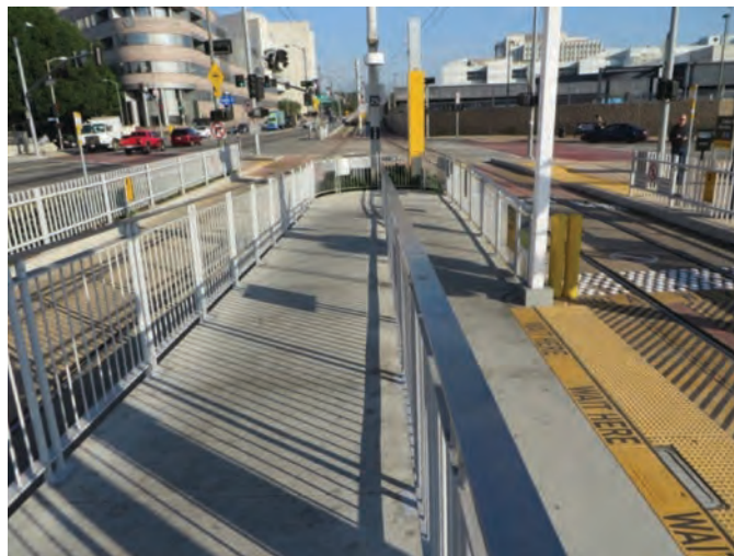
Figure 36. Extensive fencing channelizing pedestrians to the appropriate crossing.
