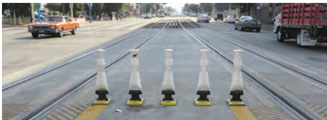
Figure 158. Bollards used to mark the edge of the crossing.
