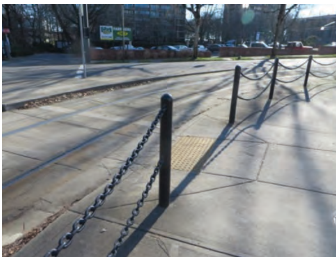
Figure 27. Example of bollards with chains used to restrict movement.
