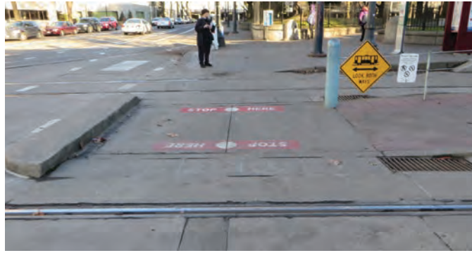
Figure 159. Raised island used to mark the edge of the crossing.
