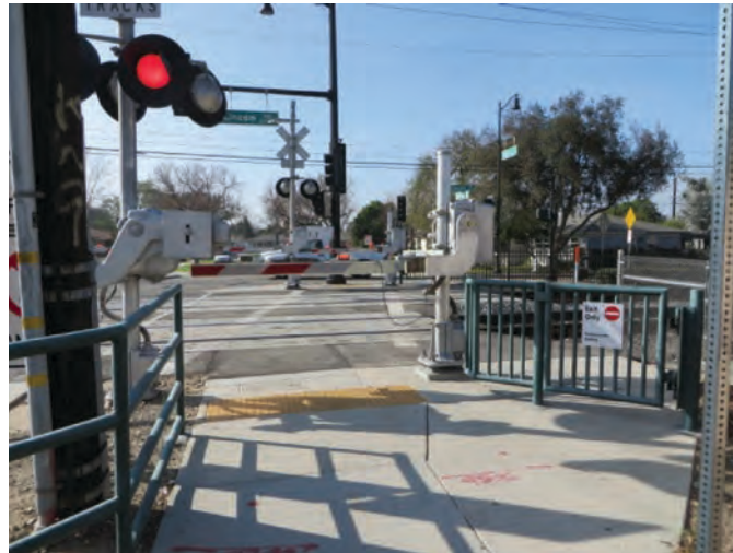
Figure 125. Example of pedestrian automatic gates with channelization and a swing gate for emergency exit.
