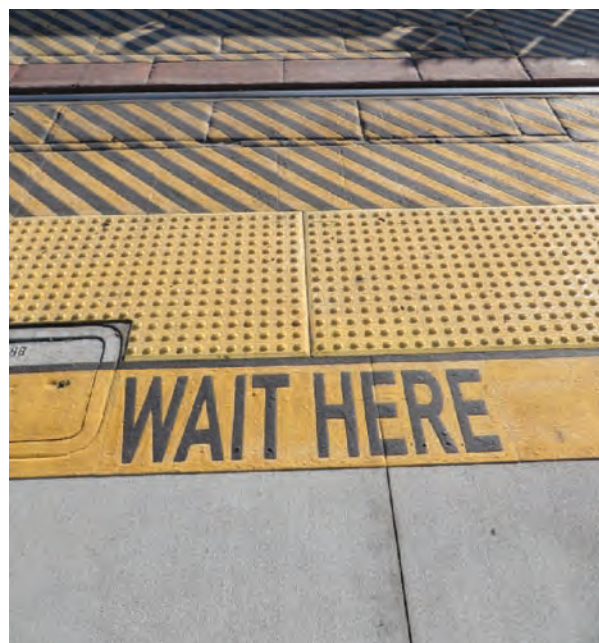
Figure 104. WAIT HERE stripe along with detectable warning and diagonal striping to indicate the dynamic envelope of train cars in Los Angeles.
