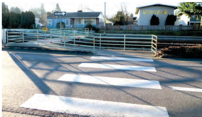
Figure 32. Example of an offset crossing.
