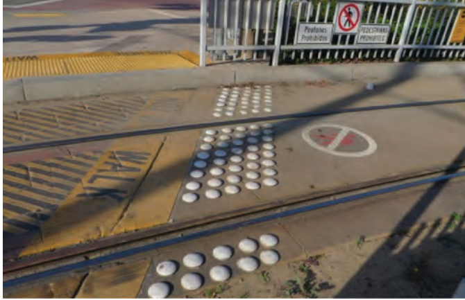
Figure 109. Symbol and word pavement markings that supplement signs indicating where pedestrians should not be walking.
