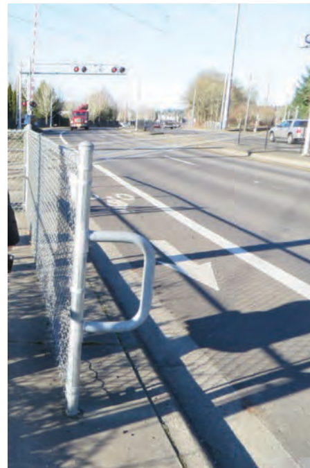
Figure 30. Example of handles used to restrict movement between the pedestrian walkway and street.
