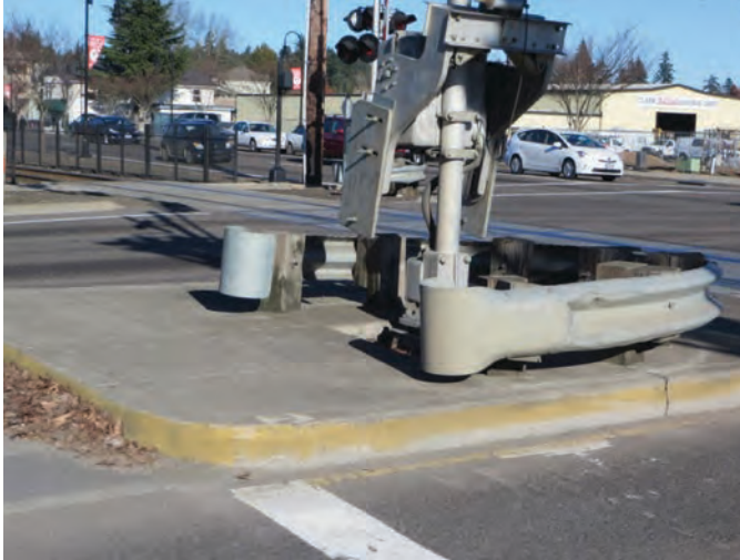
Figure 124. Barrier installed around a counterweight.
