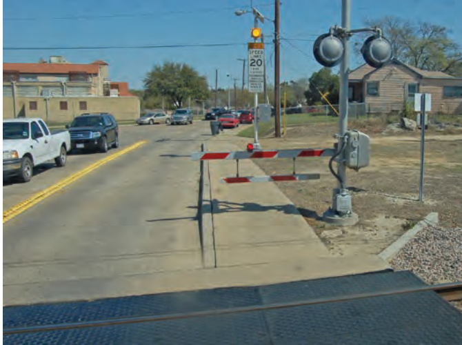
Figure 128. Example of a horizontal hanging bar on a pedestrian automatic gate at a DART crossing adjacent to a school zone.
