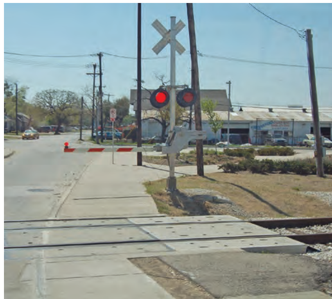
Figure 126. Example of pedestrian automatic gates without channelization.
