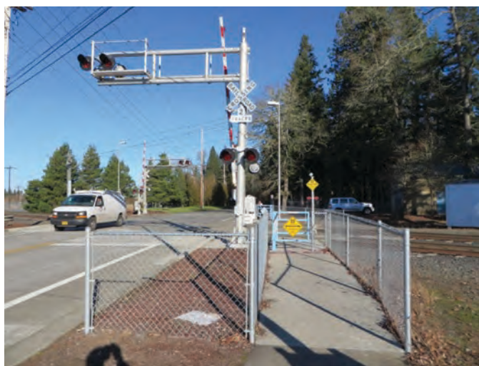
Figure 22. Example of fencing used to channelize pedestrians to appropriate crossing location.
