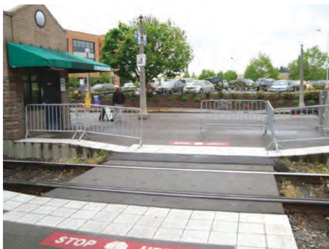
Figure 166. Gateway pedestrian channeling test using temporary barriers.
