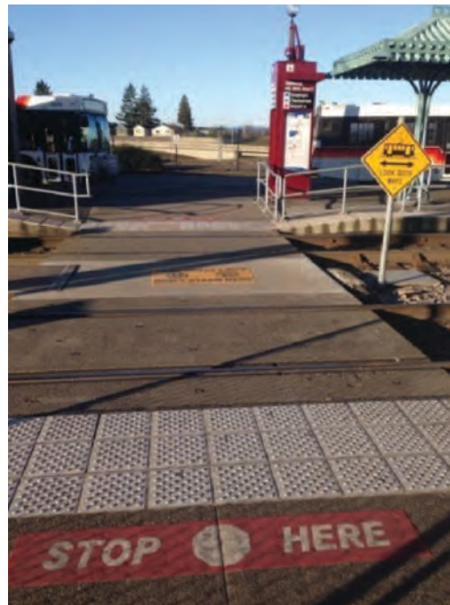
Figure 102. Example of STOP HERE pavement marking used with detectable warning at a Portland station pedestrian crossing.
