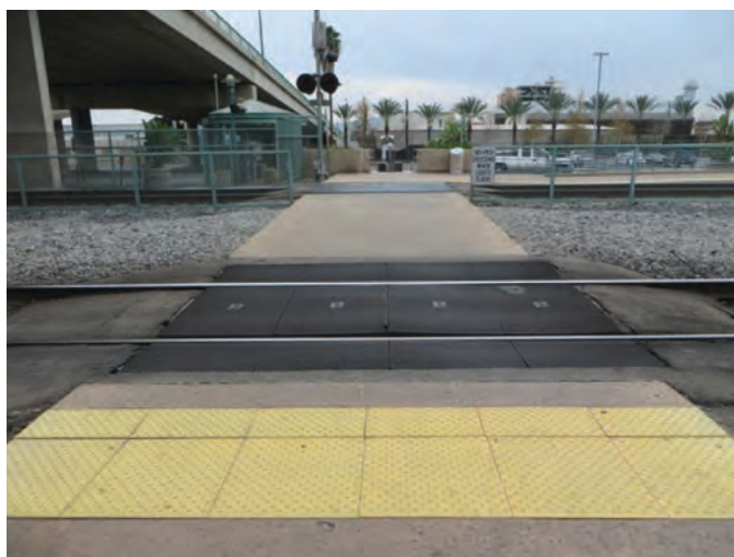
Figure 43. Example of visually contrasting surface materials, including detectable warnings, used within a clearly defined crossing surface for a pedestrian crossing within a station.
