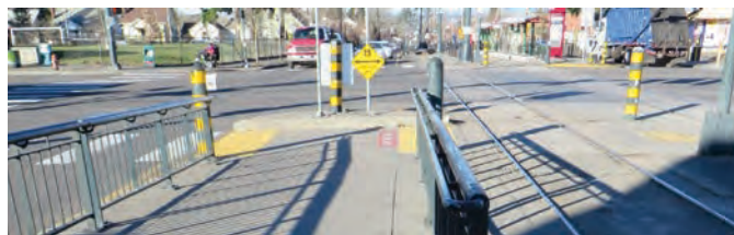
Figure 162. Several treatments used to mark the edge of the crossing, including a raised island, a sign, and bollards.
