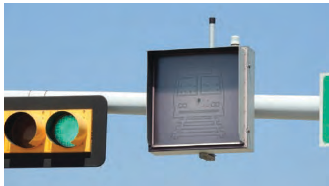
Figure 89. Example of a blank-out sign in Dallas on signal mast arm.
