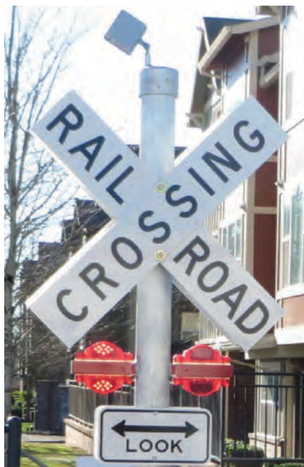
Figure 98. Closeup of a flashing-light signal assembly example installed in Portland.
