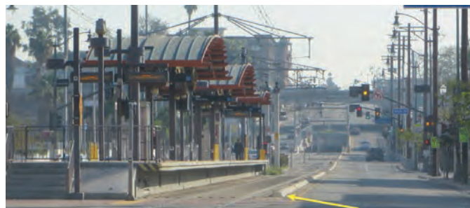
Figure 114. Example of a raised curb used alongside tracks in Los Angeles.
