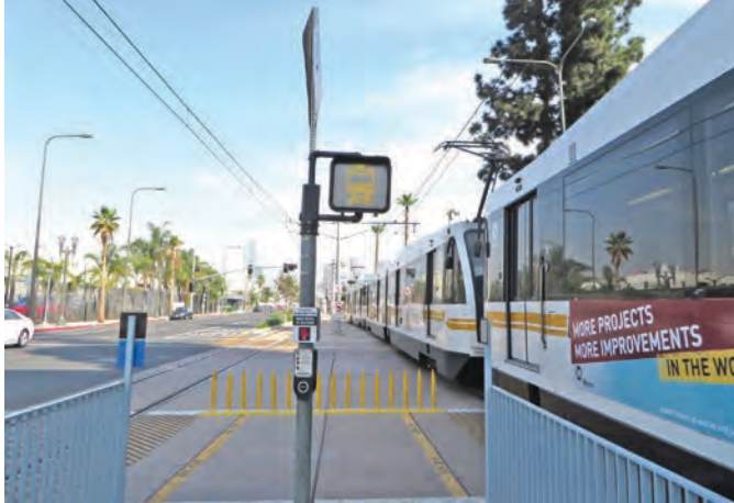
Figure 96. Example of a pedestrian push button located in a median between tracks.
