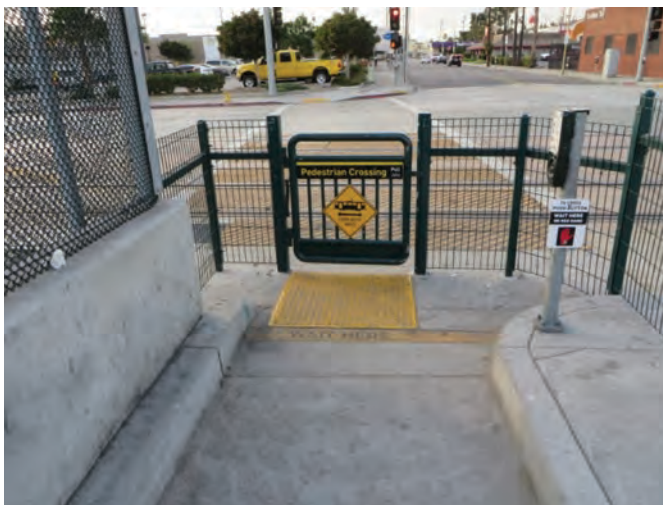
Figure 23. Fencing and curbs used to channelize pedestrians to crossing location; the photo also shows a well-located APS.
