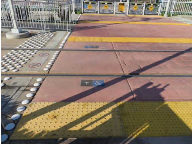
Figure 47. A smooth area within a stamped crosswalk provides an ADA-compliant surface for pedestrians in wheelchairs.
