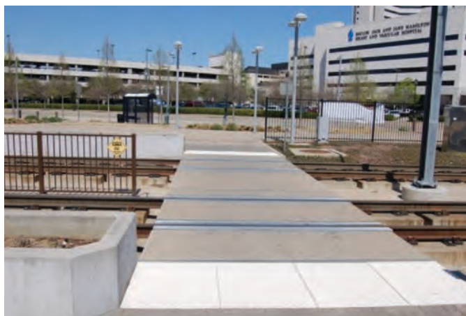
Figure 105. Example of white detectable warnings used at an in-station pedestrian-rail crossing.
