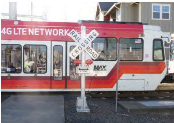
Figure 97. Flashing-light signal assembly example installed in Portland.
