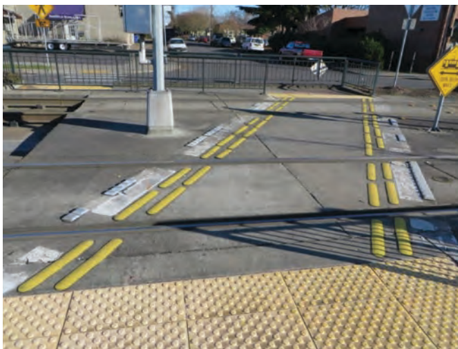
Figure 44. Three attempts to provide tactile guidance at a crossing.
