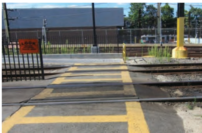
Figure 25. Example of fencing used to create a barrier to limit crossings to the paved pedestrian crossing; the fence restricts passage across the tracks within a station.
