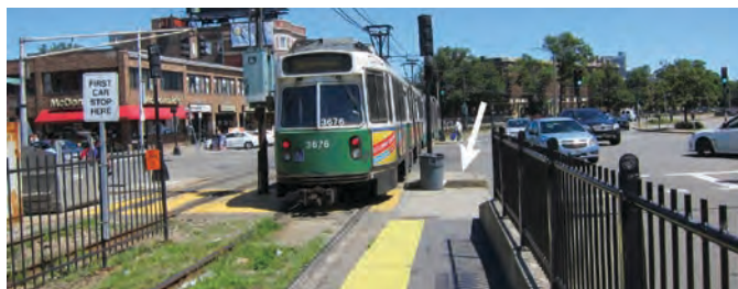
Figure 161. Raised island with a signal used to mark the edge of the crossing (trash can placed within the crossing).
