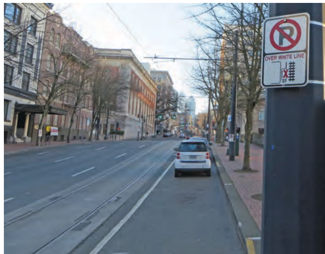
Figure 113. Example of a dynamic envelope surface treatment along with a white line between the train and parking lane.
