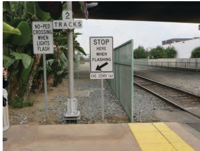
Figure 75. Example of signs used at a Los Angeles station to communicate the need to not cross when the lights are flashing and that pedestrians should stop behind the yellow detectable warning stripe.
