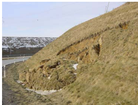
Figure 1: Slope slumping failure along roadway (Wikipedia)
