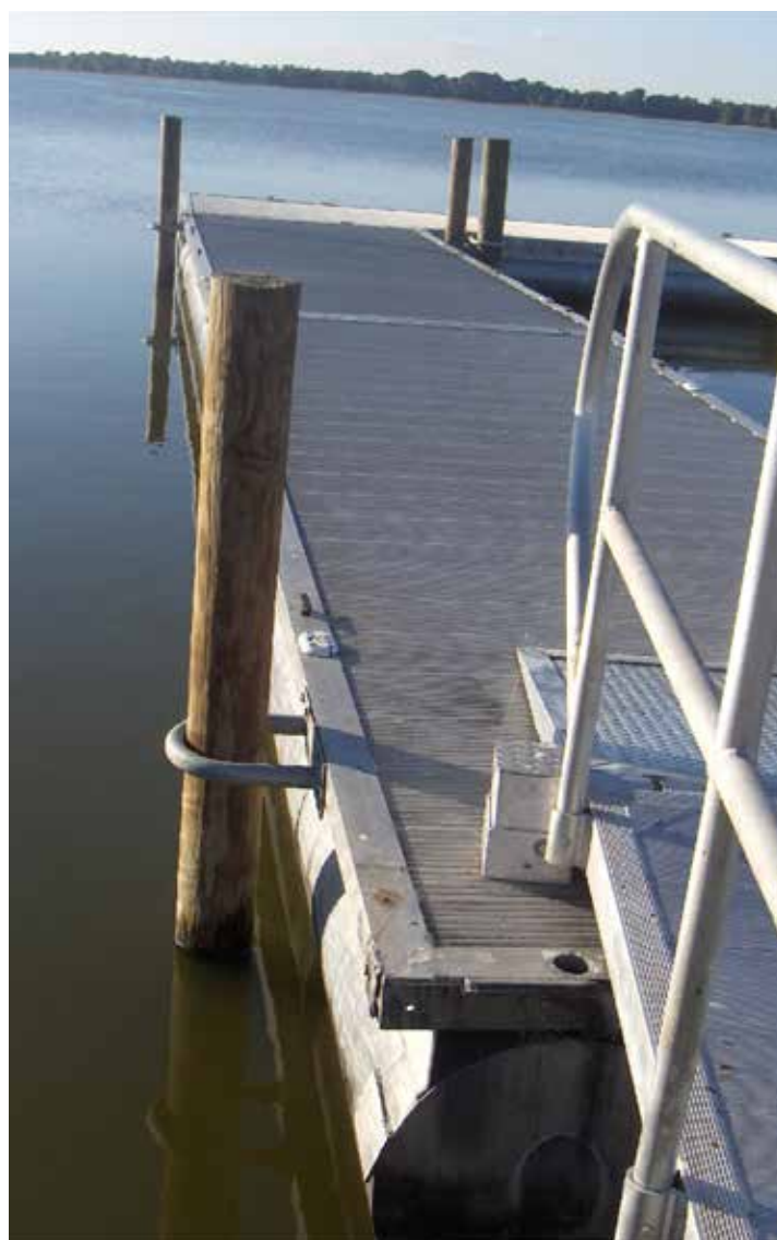
FIGURE 19 Example of a wood piling float dock attachment with spacing to accommodate a seaplane. (Credit: S. Quilty, SMQ Airport Services)
