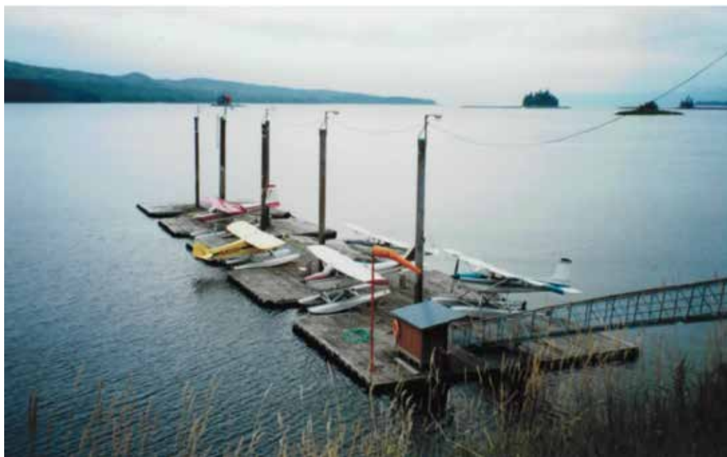
FIGURE 15 Example of floating dock with gangway, pier, and slipways. (Credit: A. Faegre 1999. Used with permission.)
