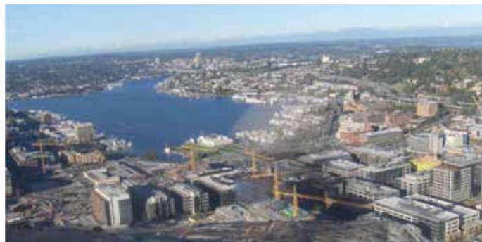
FIGURE 23 Construction cranes visible while on aircraft approach to Lake Union, Washington. (Credit: S. Quilty, SMQ Airport Services)
