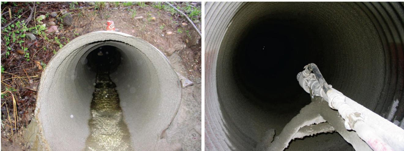
FIGURE 31 Examples of completed CSC liners (Source: Shotcrete Technologies Inc.).
