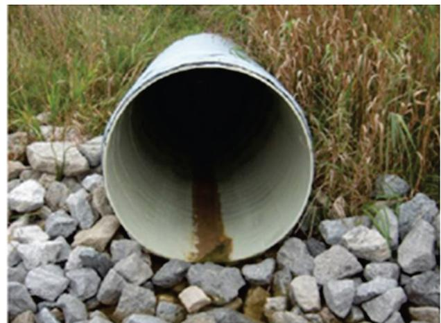
FIGURE 32 Cured-in-place pipe liner being installed and after installation in a 20-year-old corrugated steel pipe; 75-year service life assumed in design (Doherty and Angelo 2012).
