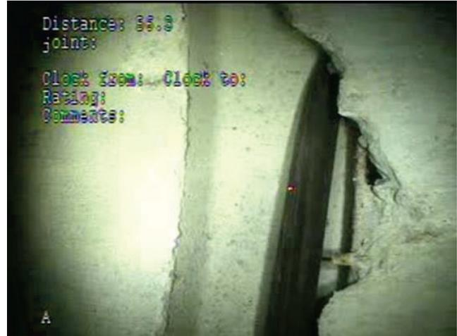
FIGURE 19 Damage at joint in RCP revealing joint sealant as detected from video inspection.
