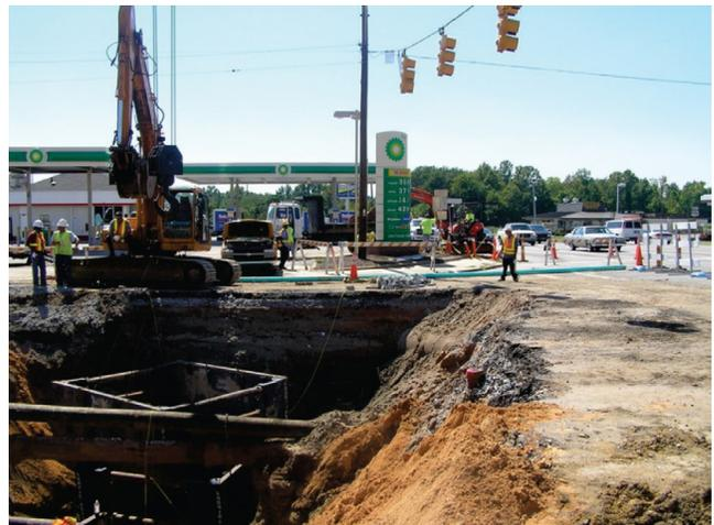
FIGURE 37 Emergency repairs following collapse of 30-in.-diameter culvert near busy intersection.
