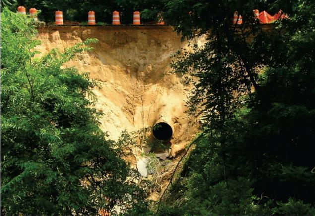
FIGURE 17 End treatment and scour failure at culvert outlet.
