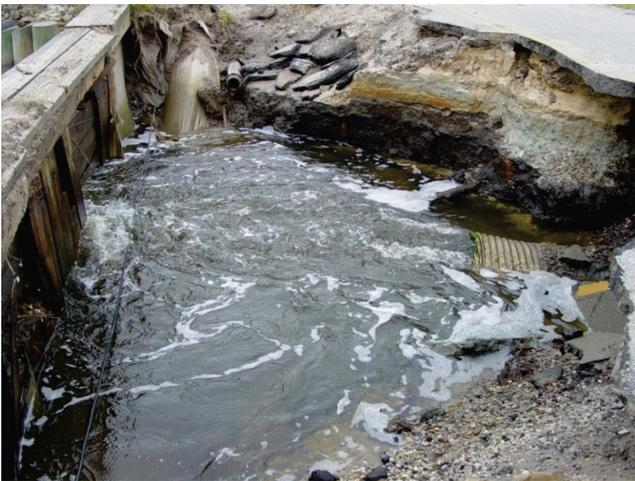
FIGURE 18 Major culvert pipe system failure behind timber headwall.
