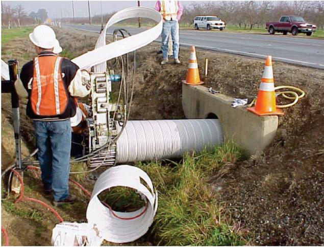
FIGURE 30 Expandable-diameter or spirally wound pipe liner being installed (Caltrans 2013).
