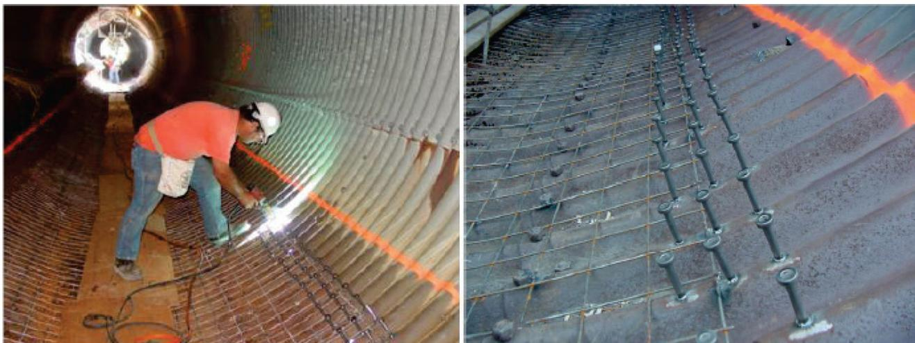
FIGURE 27 Shear connector welding studs (Nelson Studs) and wire fabric being installed prior to concrete invert paving (Caltrans 2013).
