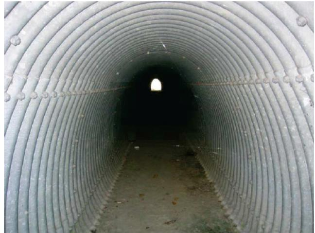
FIGURE 22 Older invert paved corrugated steel culvert in excellent condition (NYSDOT 2011).
