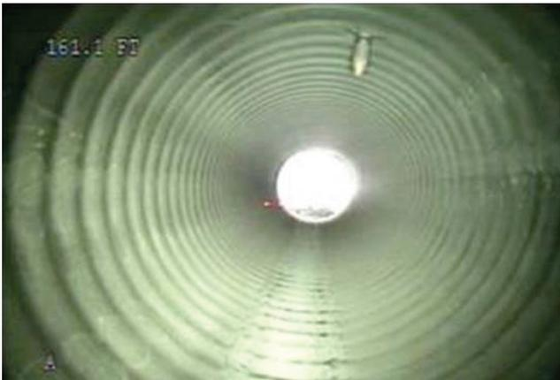
FIGURE 15 Wall penetration and puncture from metal spike.
