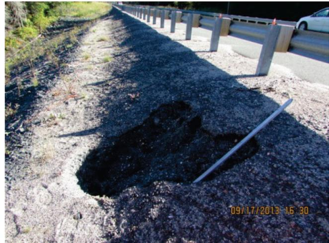
FIGURE 38 Failure of road embankment slope above a 12-ft-diameter structural plate corrugated steel culvert that had been extended at both ends. Perforation along bolt lines and 18-in. deflection at obvert of pipe.
