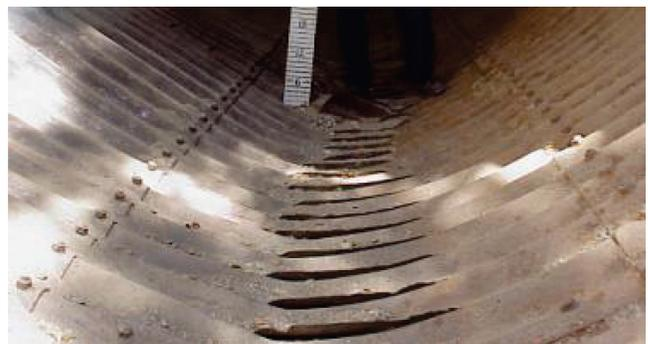
FIGURE 23 Perforated invert of metal culvert (Caltrans 2013).
