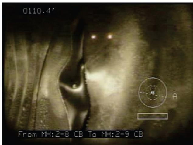
FIGURE 14 Split in inner pipe wall and local buckling.
