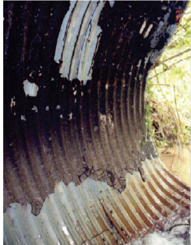
FIGURE 25 Loss of bituminous coat and paving at invert of metal pipe (Ohio DOT 2005).
