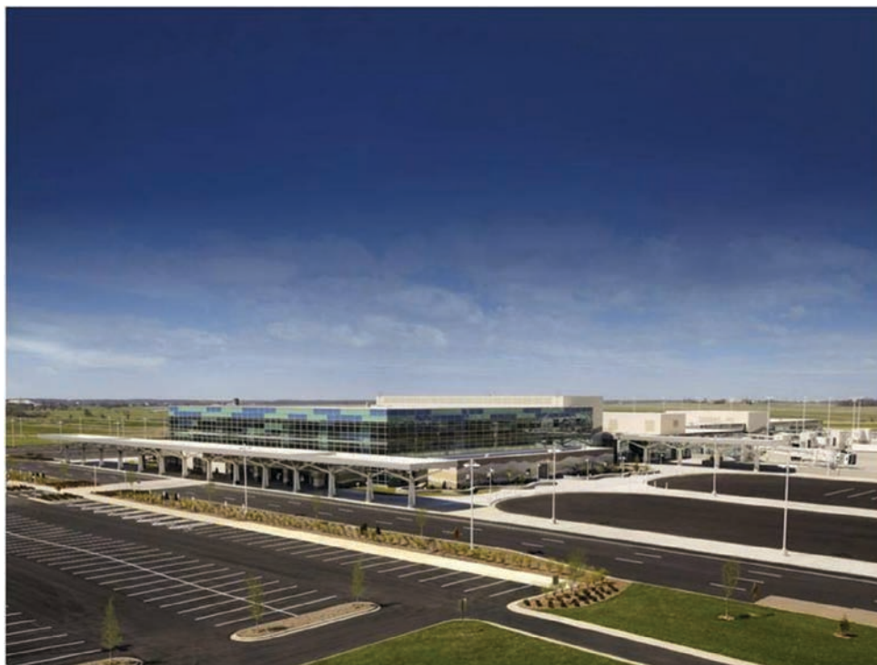
New Midfield Terminal at SGF
