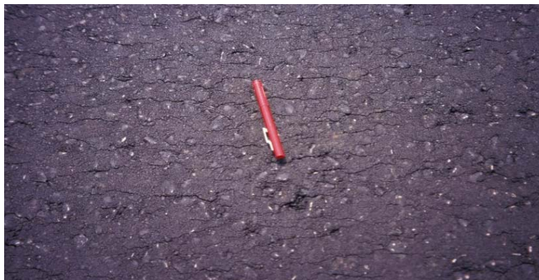
FIGURE 5 Checking of an HMA mix.
