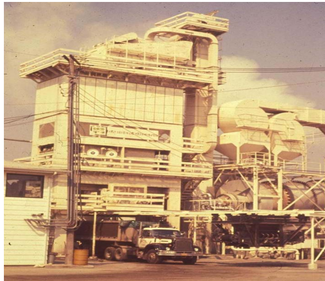
FIGURE 1 Batch plant illustration.
