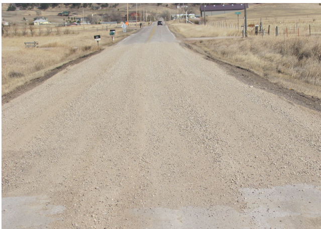
FIGURE 4 Passive conversion, a local road that has been converted to gravel surfacing only when a section fails. (Photo courtesy of K. Skorseth.)
