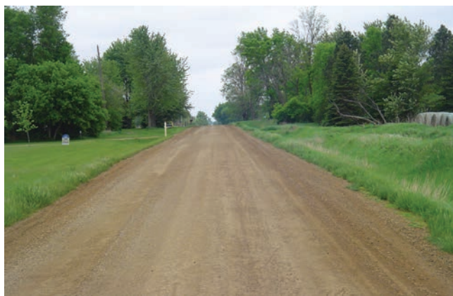
FIGURE 2 A local road that has been converted to a gravel surface. The township is able to maintain the road in acceptable condition with available funds. (Photo courtesy of K. Skorseth.)
