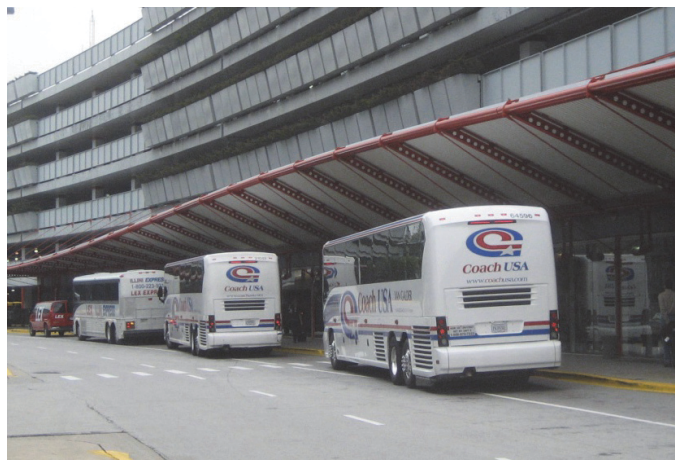
Figure 8-14. Bus center at Chicago O'Hare International Airport.
