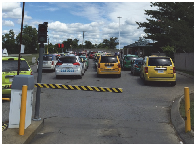
Figure 8-2. A gate controls access to the taxicab holding area at Nashville International Airport.
