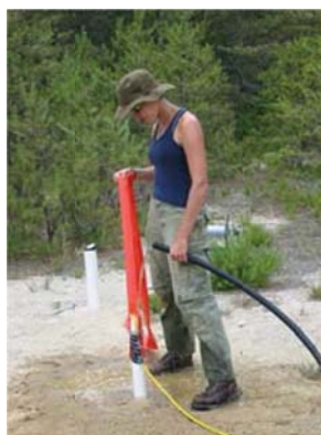
Figure Installation of a flexible borehole liner. SOURCE: USGS ( http://water.usgs.gov/ogw/bgas/toxics/FY02-MMR/gallery.html )
