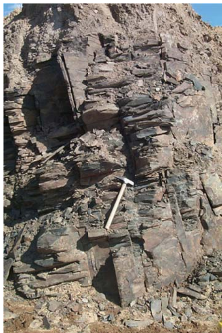
Figure 1.3 Surface outcrop of mudstone host rock for TCE contamination at the Naval Air Warfare Center Research Site in New Jersey. These fractures are controlled by bedding planes and jointing that is nearly perpendicular to bedding. SOURCE: USGS 1
