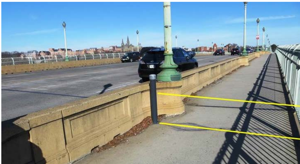
Figure 3-20. Key Bridge (Surface View)
