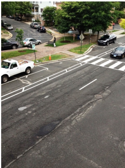
Figure 3-19. Clarendon Boulevard (Ground View)
