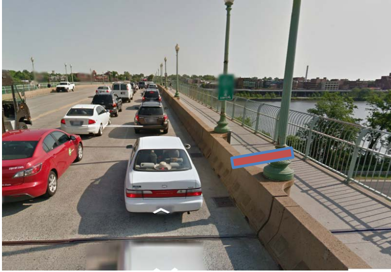
Figure 4-12. Inductive Loop Testing on Key Bridge (Washington, D.C. and Arlington, VA)
