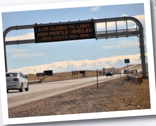
On days with high winds, Wyoming DOT closes roads to vehicles prone to being blown over.
