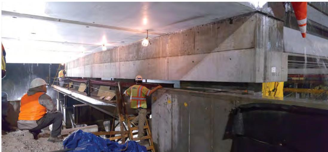
prestressed concrete beams to minimize structure depth. The new techniques from the pilot will be added to the next edition of the ABC Toolkit.
