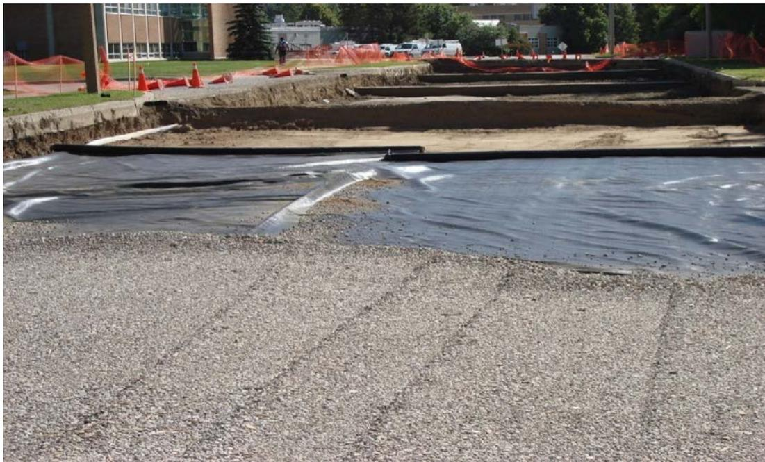
**Figure B.5. Placement of continuum recycled portland cement concrete drainage layer.**
