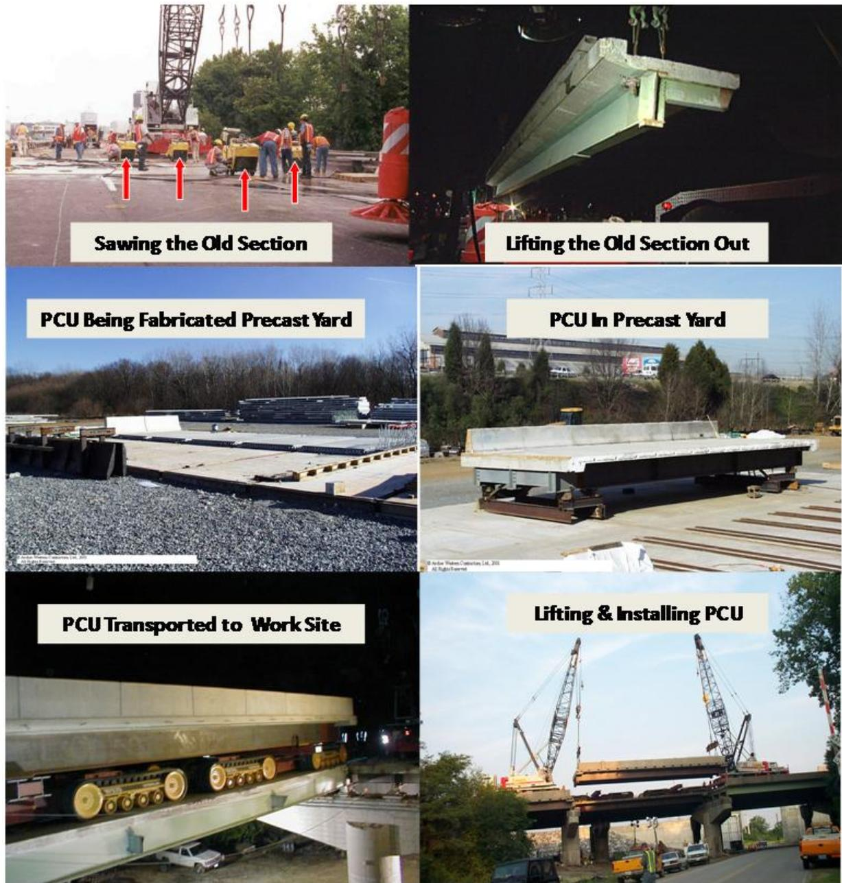
**Figure B.33. Demolition–construction sequence (3).**
