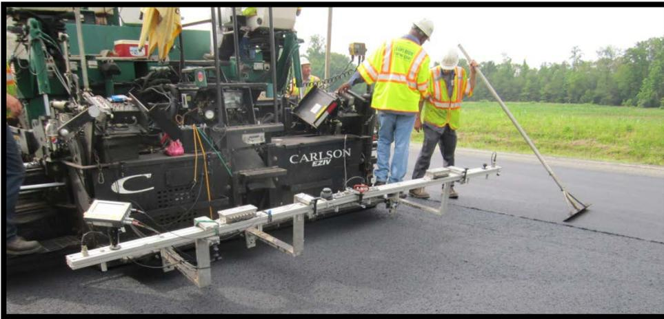
**Figure ES.1. Pave-IR collecting thermal profile.**
