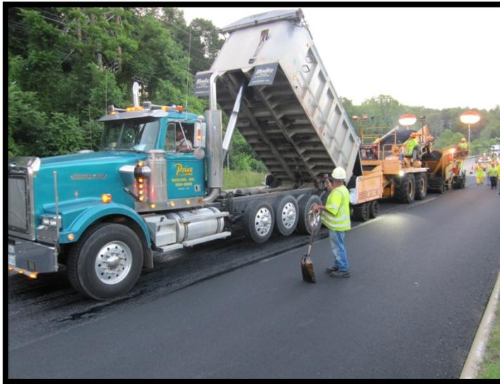
**Figure 3.1. Paving operation on US-29.**
