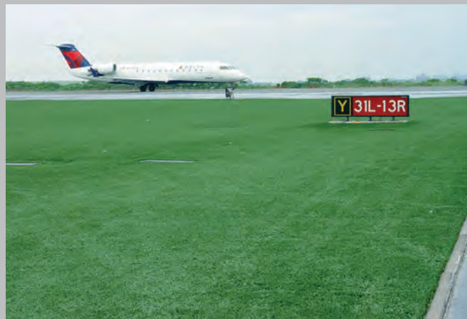
Artificial turf installed next to a runway at a northeast airport (Credit: L. Francoeur).
