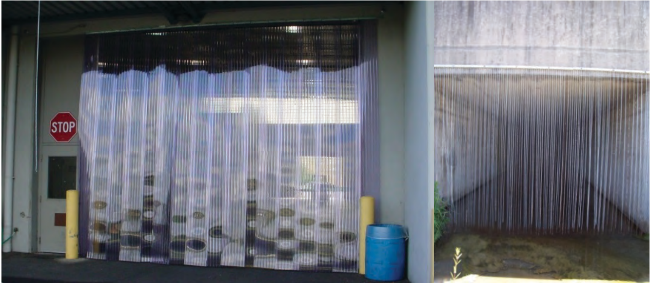
FIGURE 6 Plastic strips ( left ) and metal chains ( right ) prevent swallows and other birds from accessing protected areas attractive for nesting ( Sources : Port of Portland and H. Woods).
