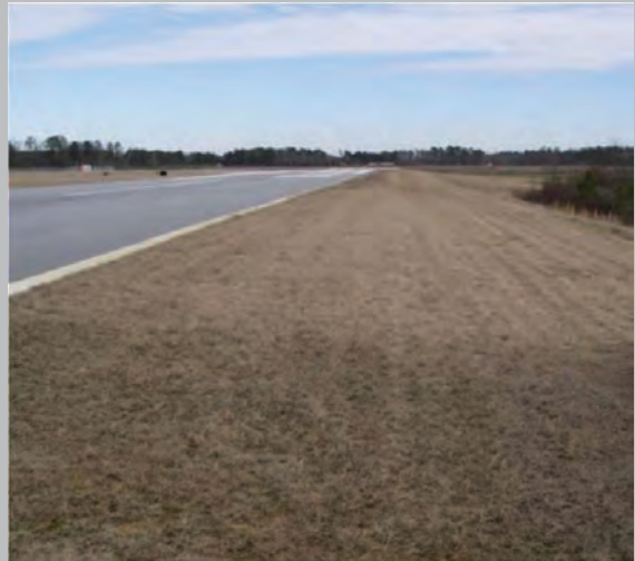
Retention ponds near airports ( left ) can now be replaced by adequate infiltration areas ( right ) (Source: NCDOT).
