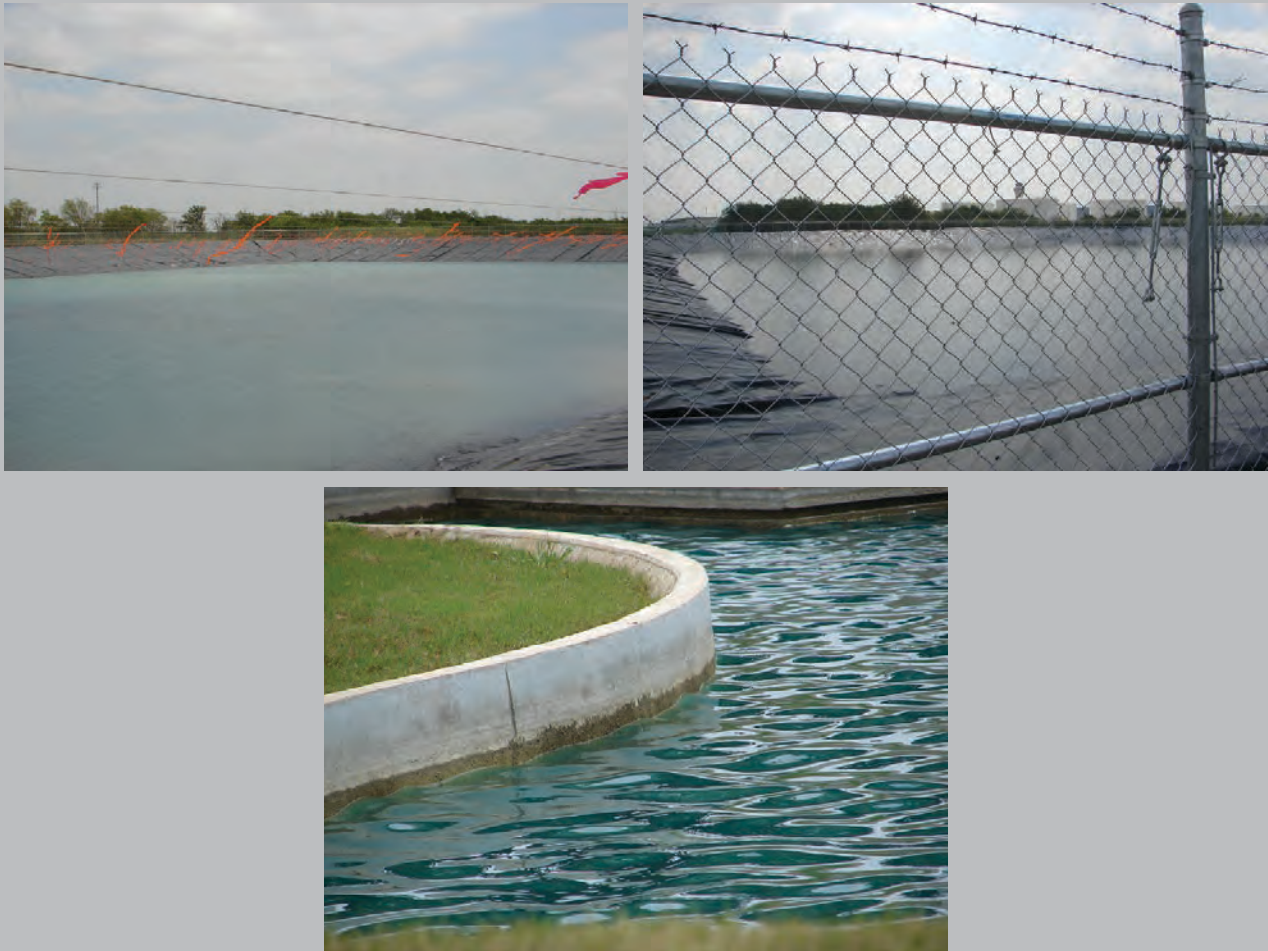
Techniques to reduce use of retention ponds by wildlife can include installing overhead cables ( top left ), fencing and impermeable substrates ( top right ), and steep walls and banks ( bottom left ) (Source: DFW).
