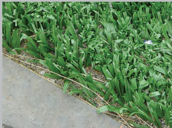
Artificial turf installed next to a runway at a northeast airport (Credit: L. Francoeur).
