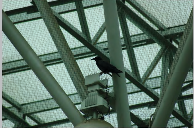
Walkway canopy at PDX ( left ) with a net preventing birds from perching on a majority of support structures ( right ) (Source: Port of Portland).
