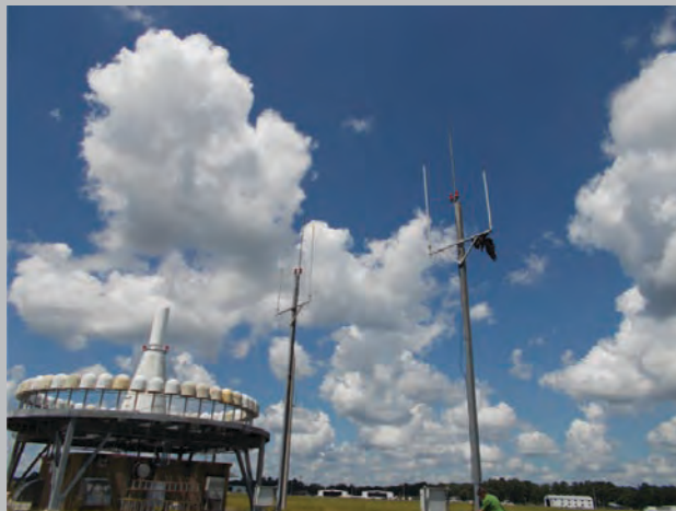
Taxidermy vulture effigy (left) hung upside-down from VOR antenna to deter vultures from perching at GNV (right) (Credit: S. Blevins).
