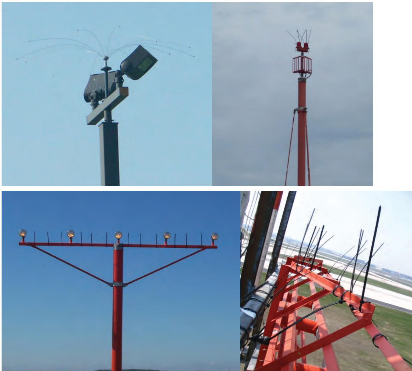
FIGURE 5 Antiperching devices on airport structures can include clockwise from top left: flexible wire set, metal spikes, and plastic cable ties in both bottom photos (Credit: H. Woods and F. Humpal).
