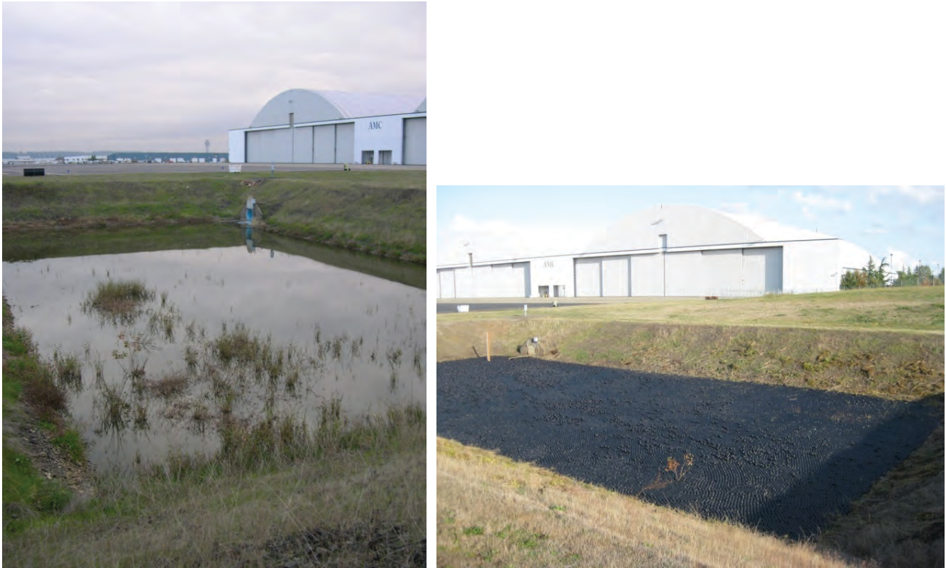
FIGURE 10 Water retention pond at PDX before and after installation of floating cover (i.e., bird balls; Source: Port of Portland). An impervious membrane was installed to maintain a water depth of 5–6 ft.
