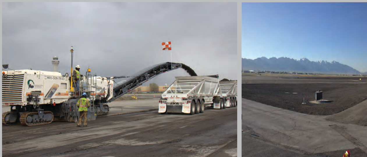
Asphalt millings left over from runway overlay projects ( left ) can be used to replace vegetation that may attract wildlife ( right ) (Source: SLC).
