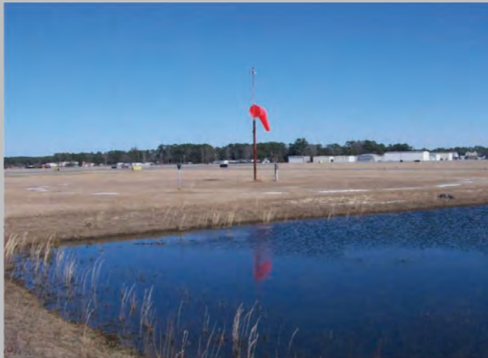
Retention ponds near airports ( left ) can now be replaced by adequate infiltration areas ( right ) (Source: NCDOT).
