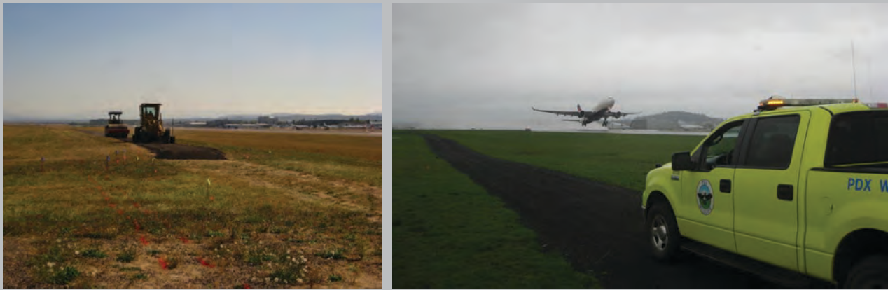
Installing roads out of asphalt millings with impervious membrane at PDX ( left ) allowed greater access to the AOA for wildlife management operations ( right ) (Source: Port of Portland).
