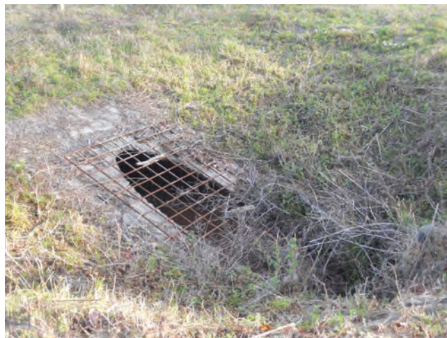
FIGURE 7 Covering over a culvert to prevent use by wildlife ( Source : A. Johnson).
