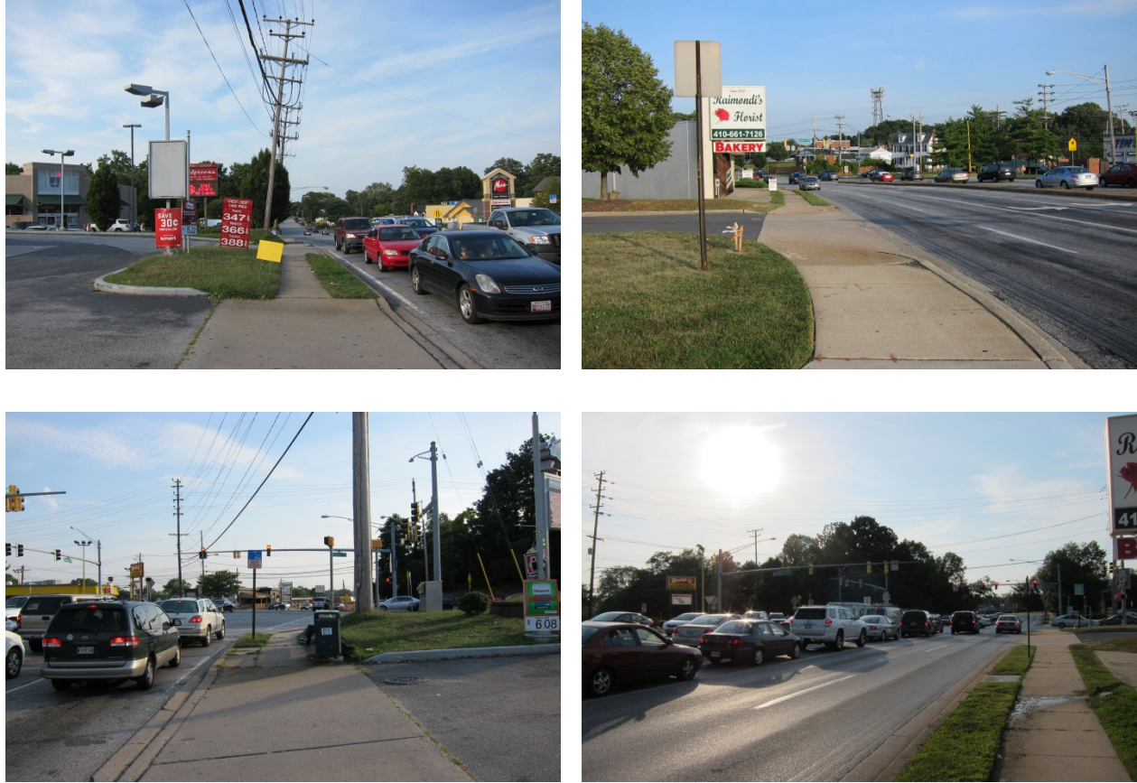
Figure 2.7. MD 147 at Joppa Road.
