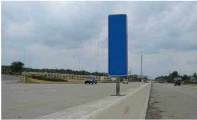
(a) Top plate-mounted sleeve and perforated square tube support
