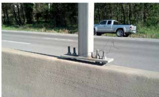
(d) Top-mounted base plate with structural square tube support
