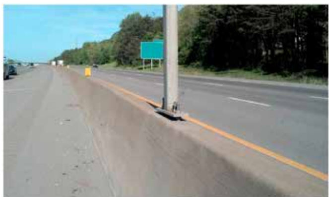
(d) Top-mounted base plate with structural square tube support
