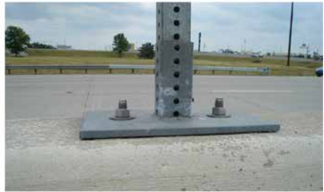
(a) Top plate-mounted sleeve and perforated square tube support
