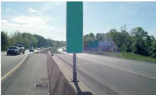
(b) Top plate-mounted angle and perforated square tube support
