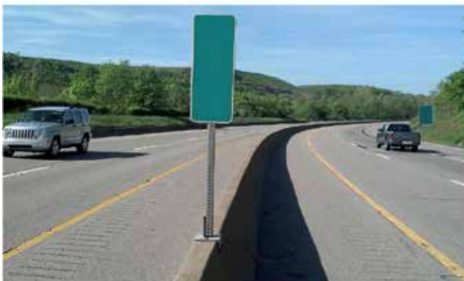
(c) Adjustable angle-mounted angle and perforated square tube support
