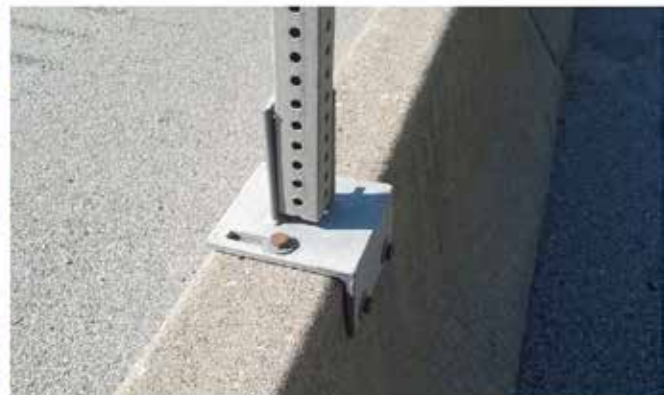
(c) Adjustable angle-mounted angle and perforated square tube support
