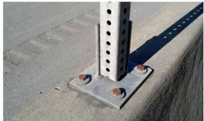
(b) Top plate-mounted angle and perforated square tube support
