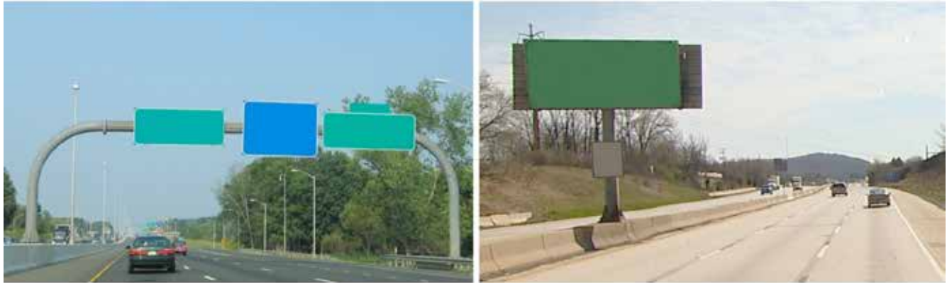
(a) Single pipe overhead sign supports
