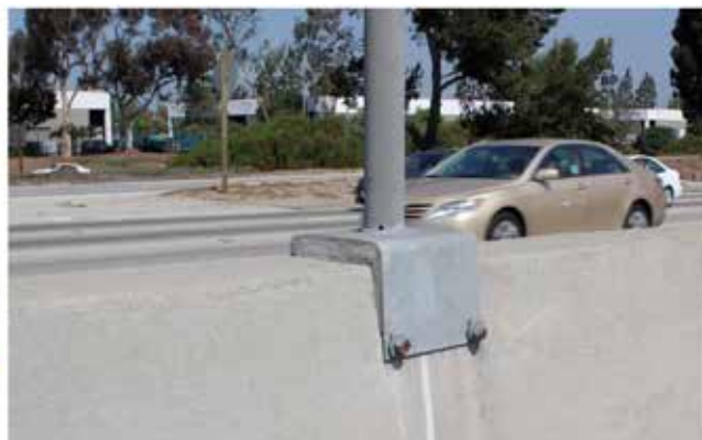
(b) Saddle base plate support
