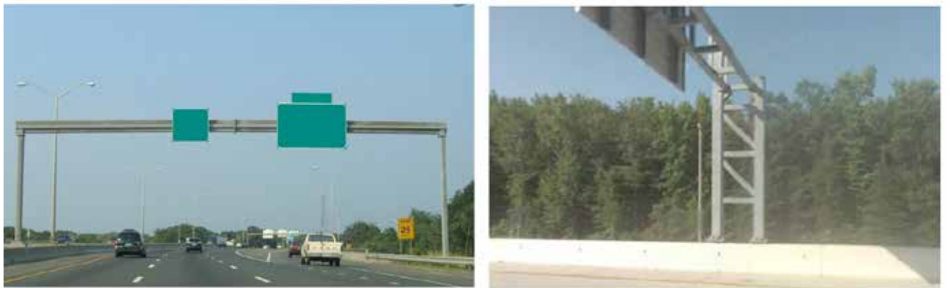
(c) Structural square tube vertical supports
