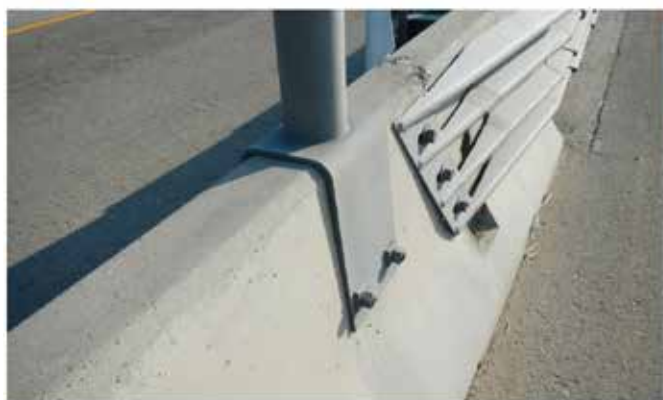
(c) Saddle base plate with round pipe supports
