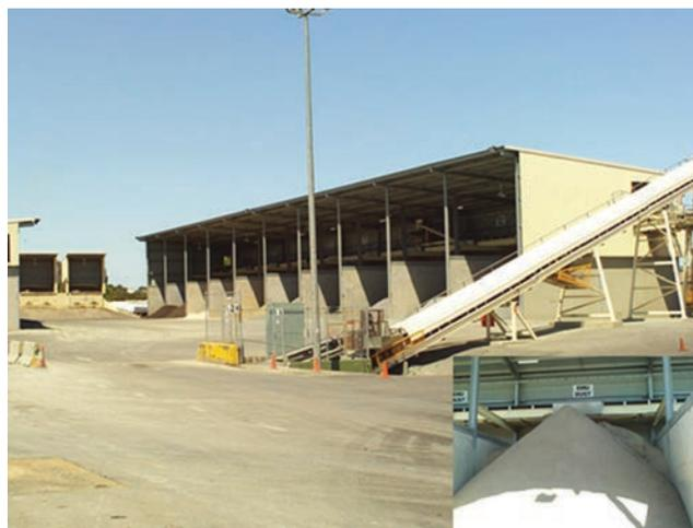
FIGURE 7 Storage shed for aggregate stockpiles. (Source: Randy West, NCAT.)
