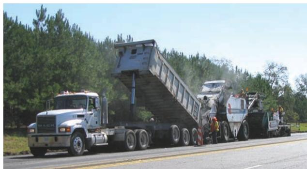
FIGURE 9 Paving operation with use of MTV. (Source: Don Watson, NCAT.)
