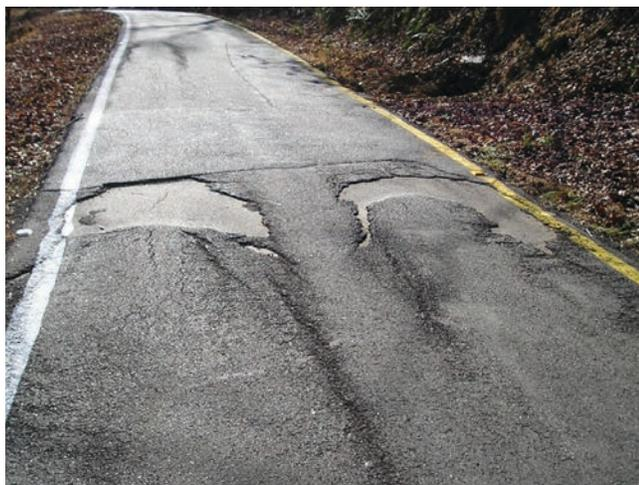
FIGURE 8 Slippage of thin overlay. (Source: Don Watson, NCAT.)
