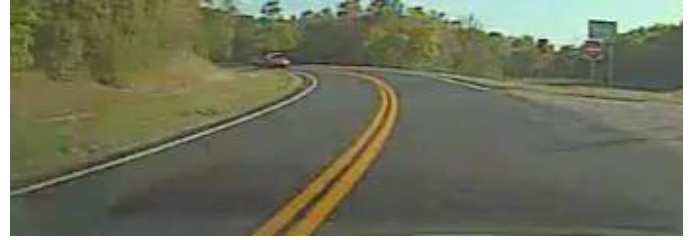
Pavement condition indicated as “normal.”
