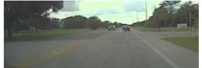
Pavement condition indicated as “moderate.”
