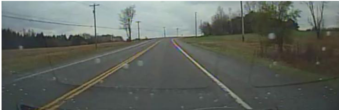
Moderate roadway furniture.
